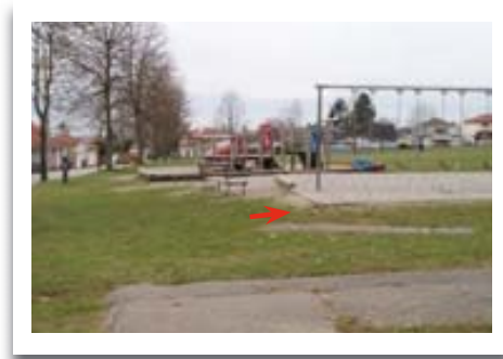
Bench is not located on accessible surface and there is no path to reach it. PHOTO COURTESY OF SHIRA STANDFIELD
