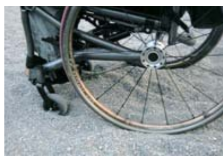
Inaccessible safety surface - pea gravel. PHOTO COURTESY OF SHERRY CAVES
