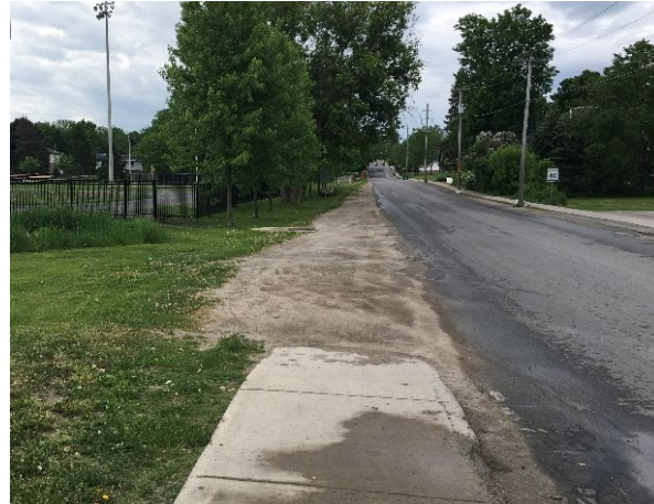
Figure 22. The sudden end of this sidewalk is an example of a connection gap in the hamlet of Sydenham, South Frontenac Township.
