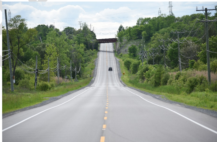
Figure 15. Paved shoulders on Rutledge Road in South Frontenac.
