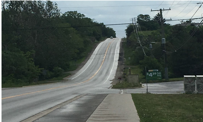
Figure 18. Sidewalk and raised cycle track end transitioning to paved shoulder in Sydenham.
