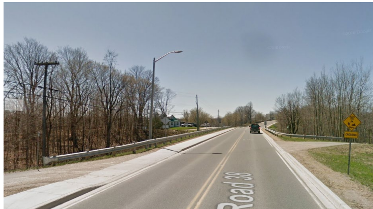
Figure 35. Angled crossing of the Tay Havelock Trail over Road 38 in Sharbot Lake. Motorized vehicles are allowed (Google).
