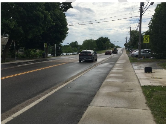
Figure 11. A raised cycle track in the village of Sydenham (South Frontenac Township).
