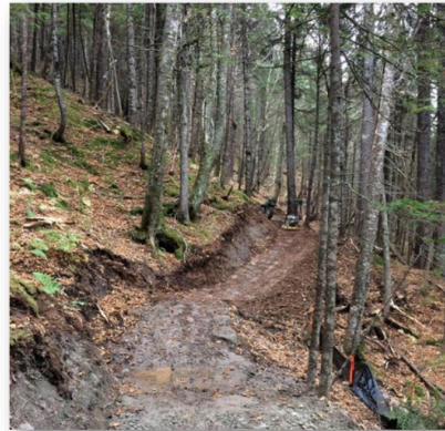
Machine built, Single Track 1.5-2 meters
