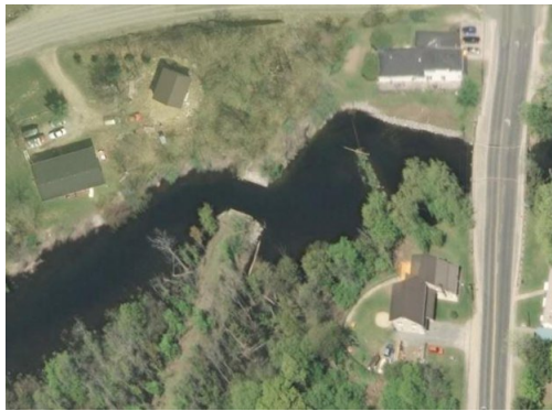
Figure 1 K&P Trail Bridge at Verona 2008
