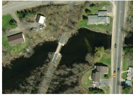
Figure 2 K&P Trail Bridge at Verona 2014
