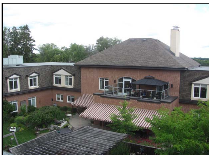
Photo No. 8: West elevation of east wing
