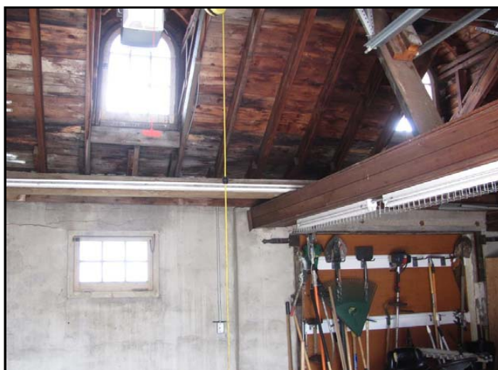
Photo No. 6: Garage interior view of east wall
