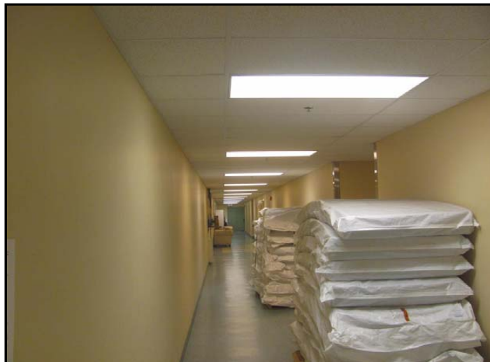
Photo No. 31: Basement corridor
