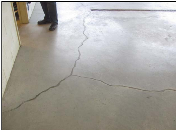
Photo No. 3: Cracks filled in slab-on-grade
