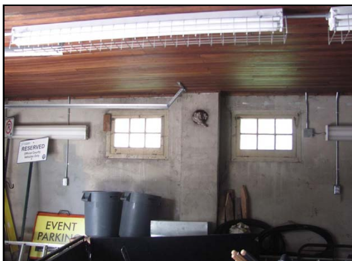
Photo No. 4: Garage interior view of north wall
