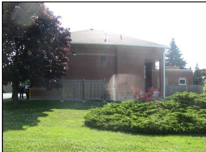
Photo No. 6: West elevation
