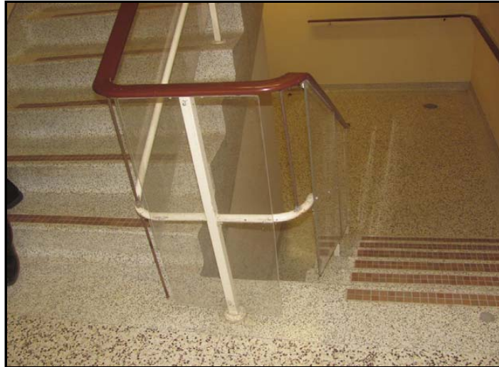
Photo No. 33: 1968 stairwell
