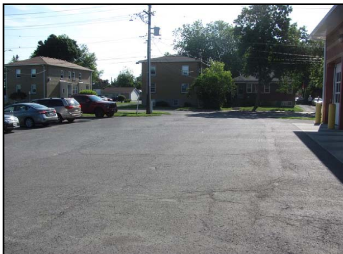
Photo No. 26: Paving at north
