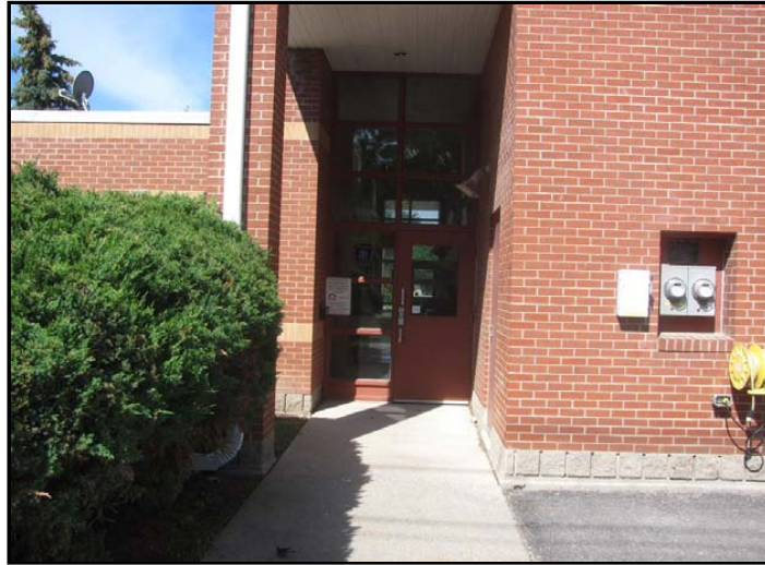
Photo No. 9: East entrance door
