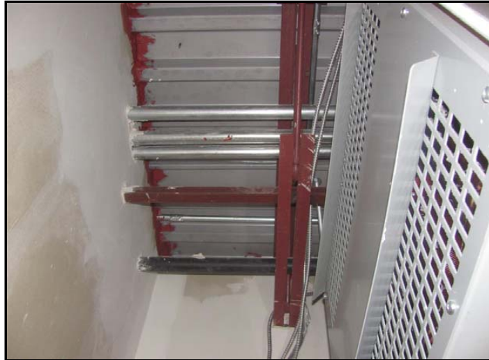
Photo No. 3: Steel roof structure at 2004 addition
