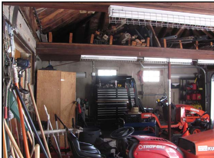
Photo No. 5: Garage interior view of south wall
