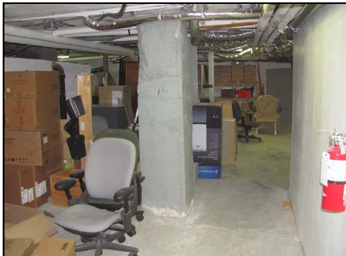
Photo No. 5: Concrete column in basement
