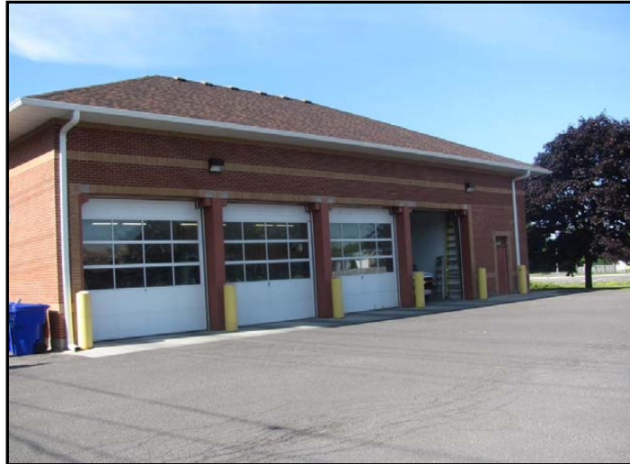
Photo No. 5: North elevation
