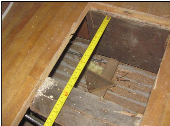
Photo No. 3: Wood floor joists seen in attic
