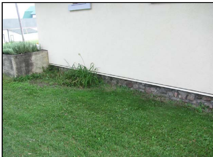
Photo No. 8: Exposed foundation wall for shed
