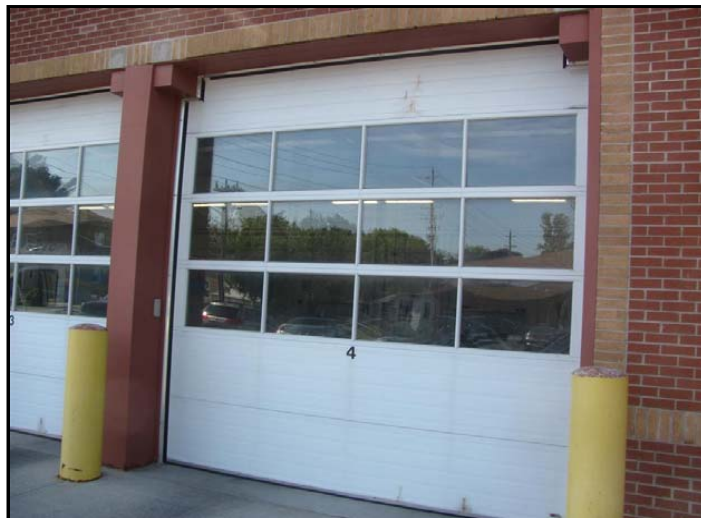
Photo No. 10: Typical overhead door
