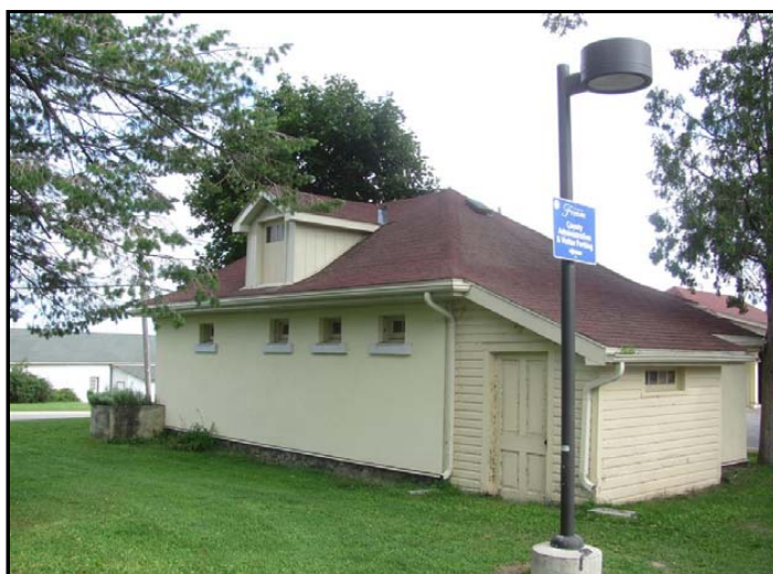
Photo No. 12: Shed north elevation
