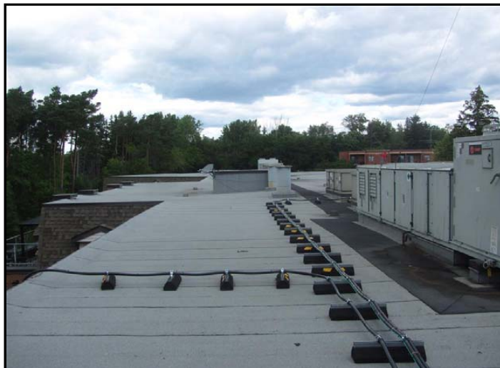
Photo No. 15: Main roof level above west wing
