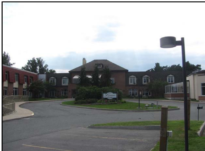
Photo No. 1: Fairmount Home street view
