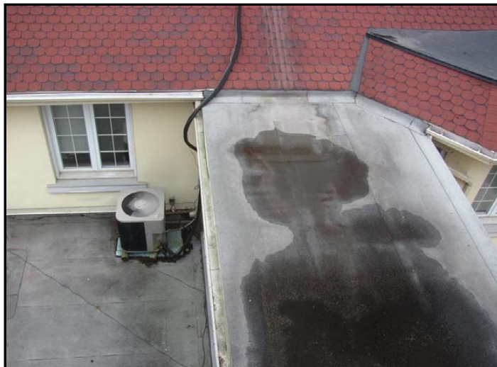
Photo No. 15: Modified bitumen flat roofing
