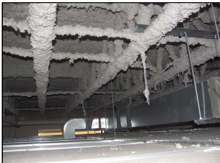
Photo No. 2: Concrete-topped steel deck ground floor structure at 1968 wing
