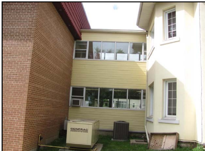
Photo No. 11: Link south elevation
