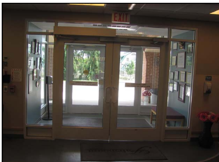
Photo No. 14: Main entrance doors
