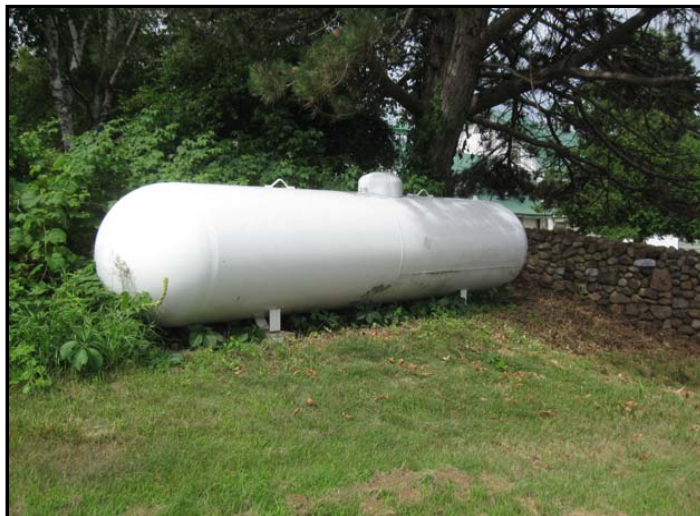
Photo No. 23: Propane storage tank
