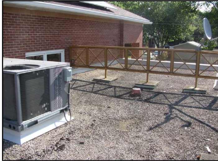
Photo No. 11: Flat roof at south
