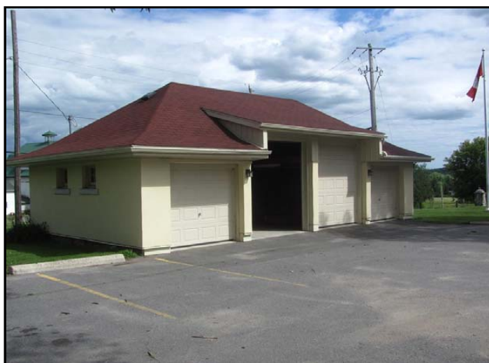
Photo No. 10: Garage west elevation
