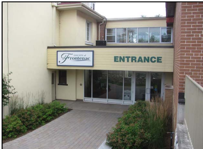
Photo No. 9: Link north elevation
