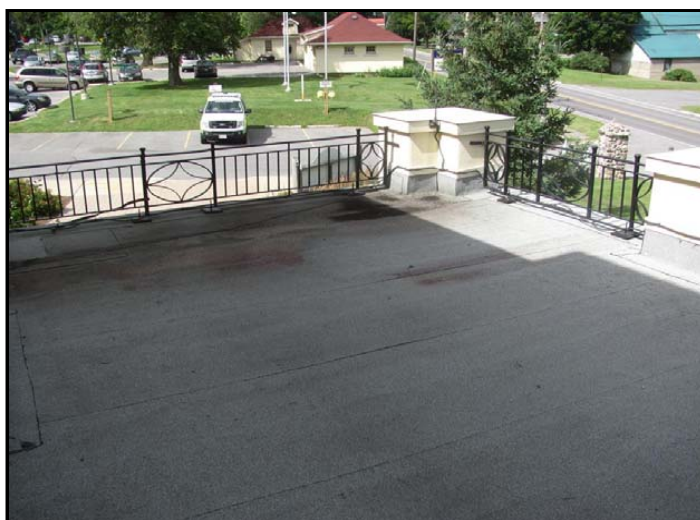
Photo No. 16: Terrace roof
