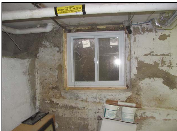
Photo No. 6: Concrete foundation wall
