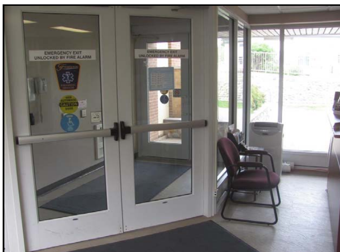
Photo No. 14: Reception entrance doors
