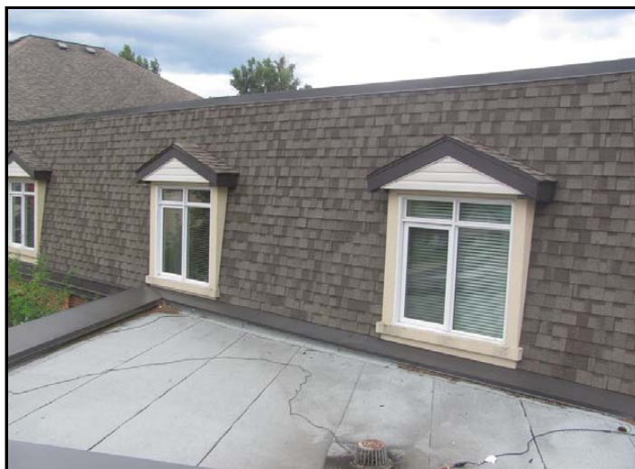
Photo No. 18: Asphalt-shingled mansards
