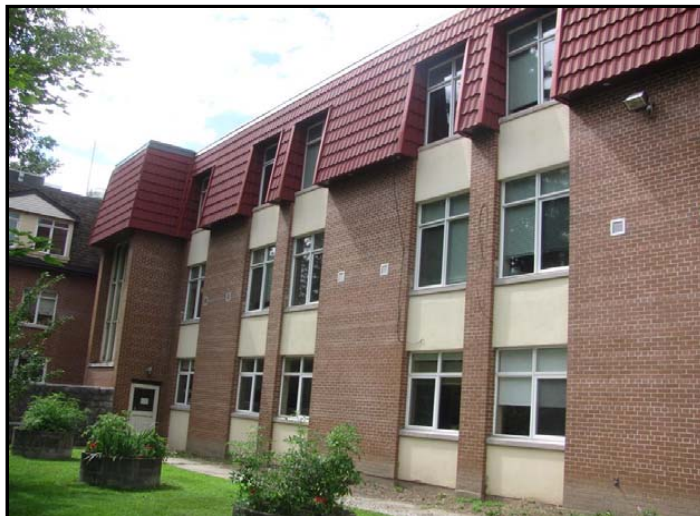
Photo No. 7: South elevation of 1968 wing
