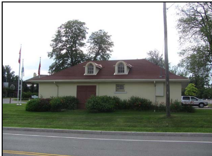
Photo No. 1: Garage viewed from street
