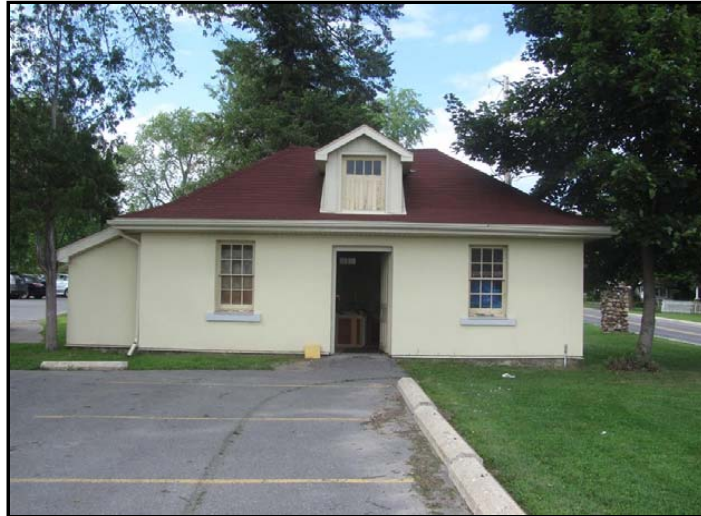
Photo No. 13: Shed south elevation
