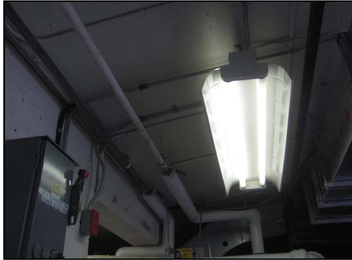
Photo No. 5: Sloped concrete roof structure at Auditorium
