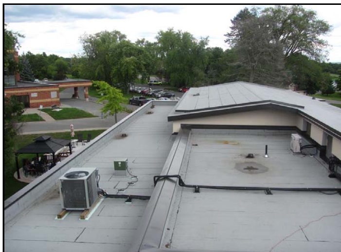
Photo No. 16: Auditorium roof
