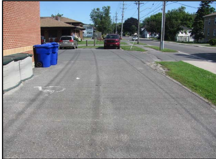
Photo No. 27: Paving at east
