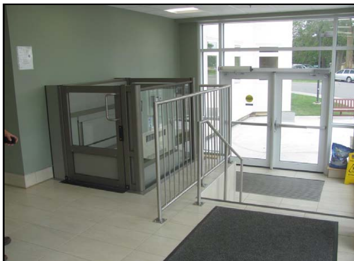
Photo No. 36: Auditorium vestibule
