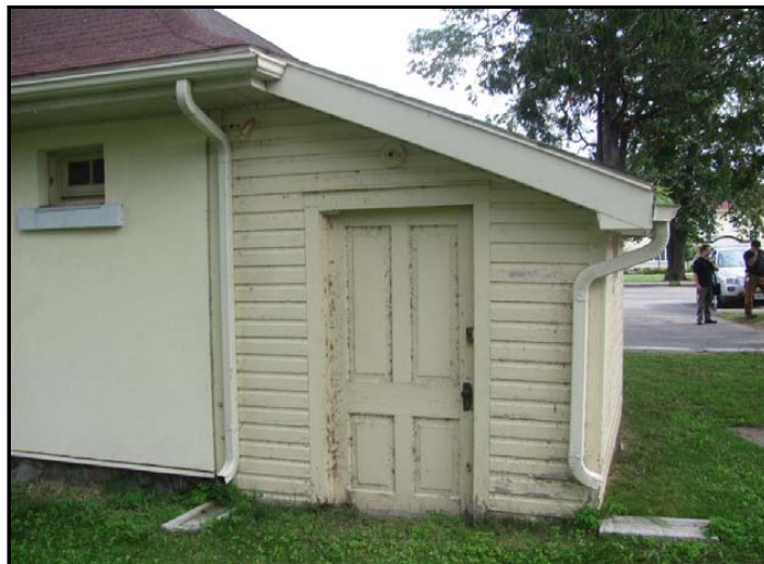
Photo No. 14: Shed enclosed storage room addition
