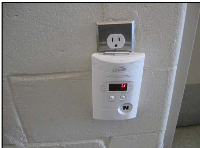
Photo No. 14: Residential style CO detector
