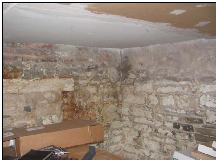
Photo No. 4: Stone rubble and masonry foundation wall
