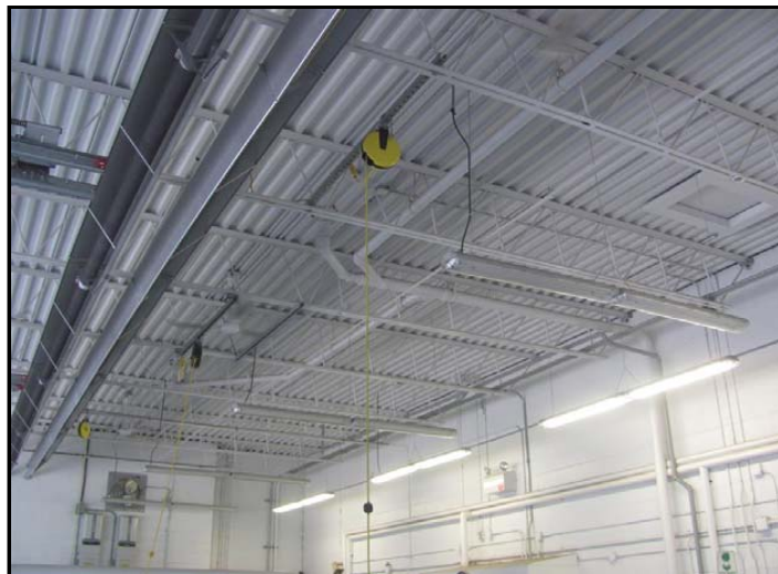
Photo No. 2: Steel-framed roof deck
