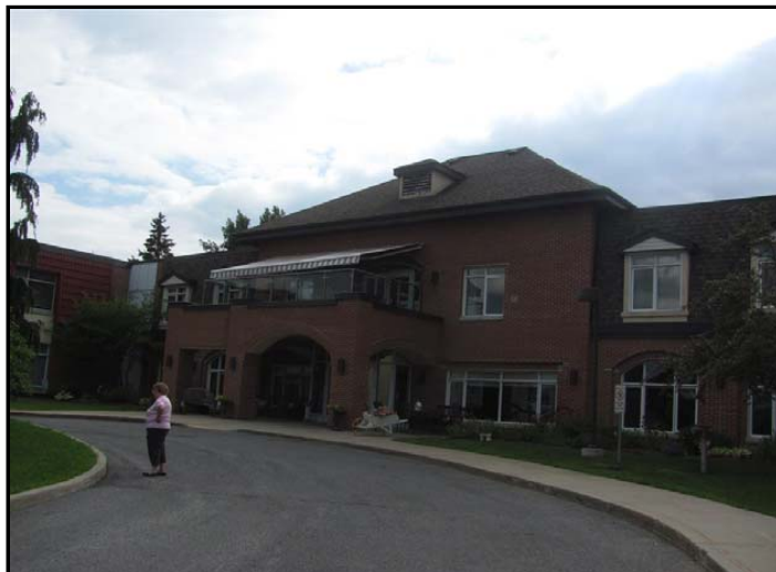
Photo No. 9: East elevation of east wing
