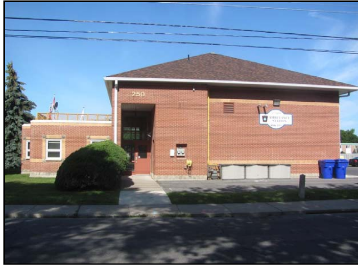
Photo No. 1: Street view of the east elevation
