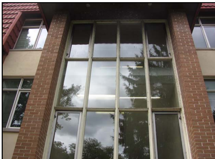
Photo No. 12: 1968 stairwell windows
