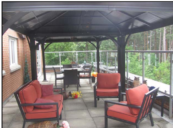
Photo No. 6: Balcony on west elevation of west wing
