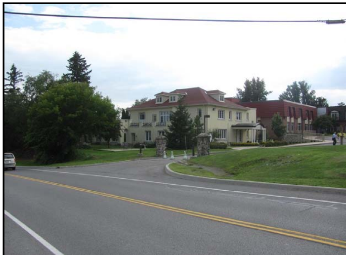
Photo No. 1: Old House street view
