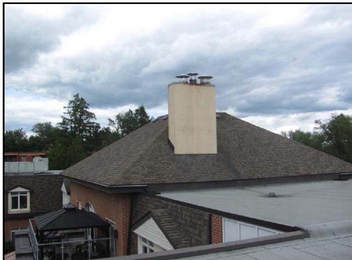
Photo No. 17: Centrally-located sloped roofing
