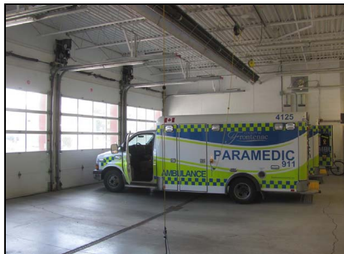
Photo No. 18: Garage finishes
