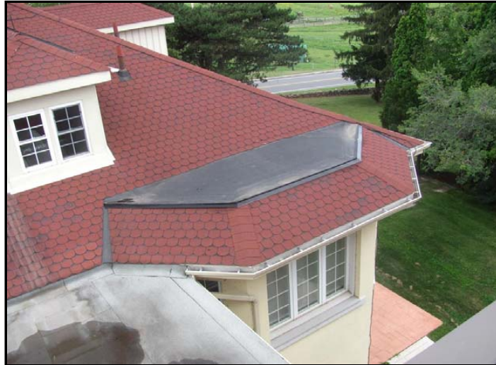
Photo No. 17: EPDM flat roofing
