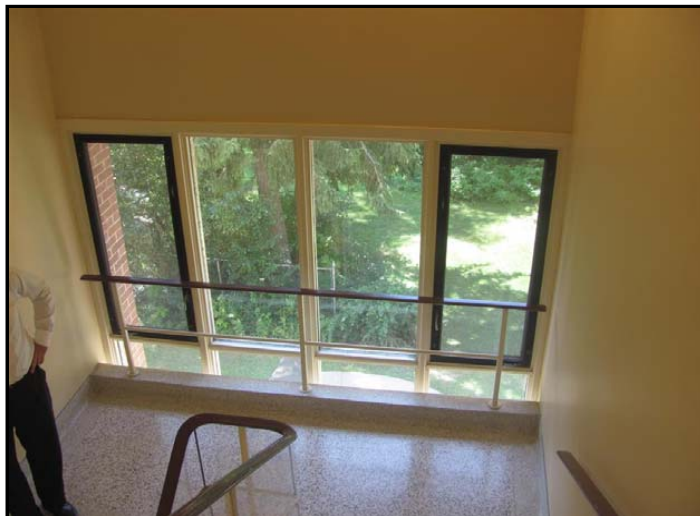
Photo No. 13: Stairwell S2 guard
