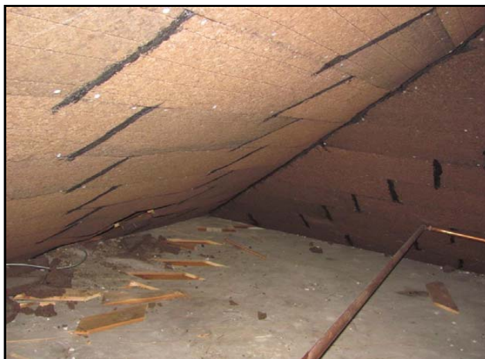
Photo No. 10: Cork insulation at attic
