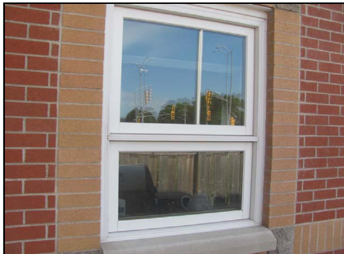
Photo No. 8: Typical window
