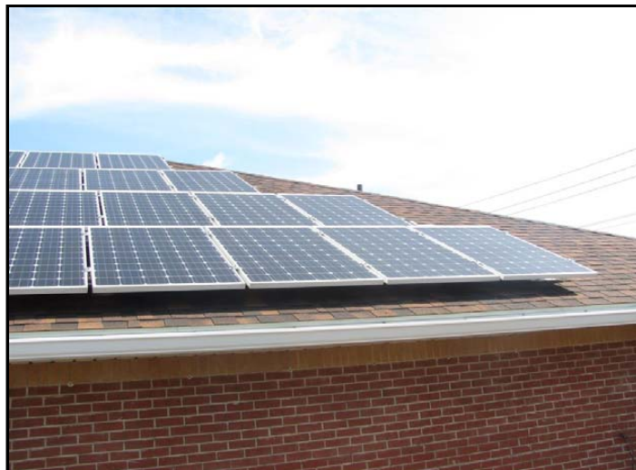
Photo No. 12: Sloped roofing
