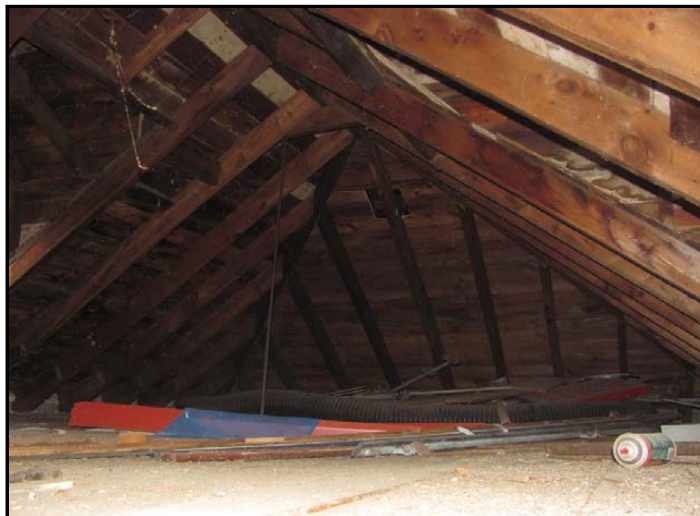
Photo No. 9: Shed's attic
