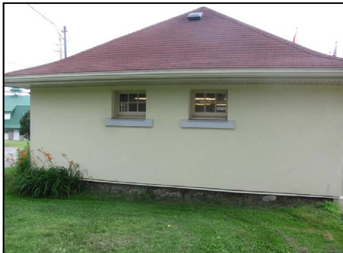
Photo No. 11: Garage north elevation
