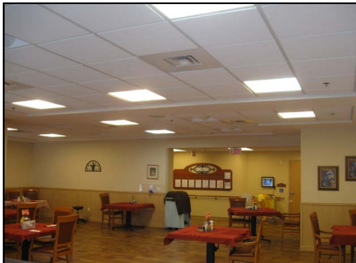
Photo No. 59: Dining room lighting
