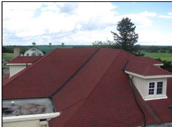
Photo No. 18: Asphalt shingle roofing
