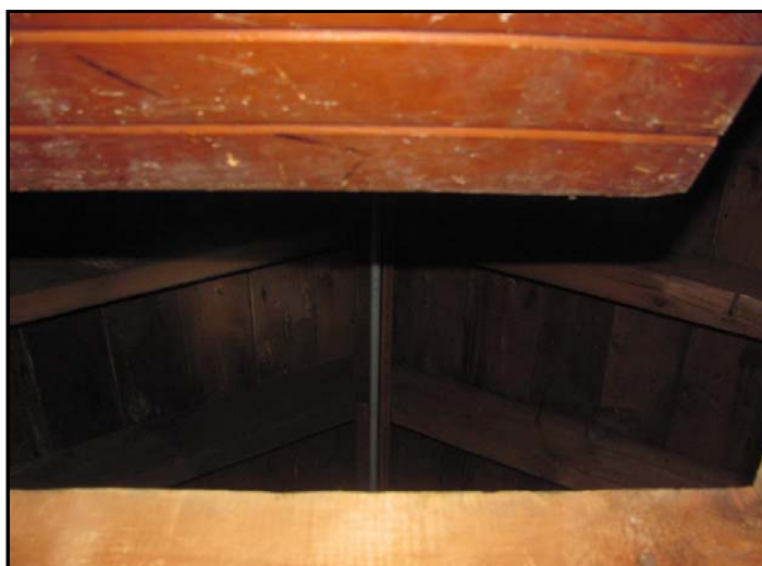
Photo No. 2: Plank sheathing on wood rafters in attic
