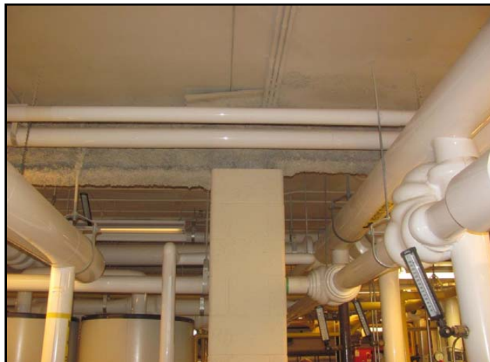
Photo No. 4: Precast ground floor structure at 2004 addition
