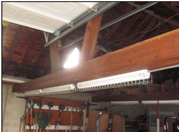
Photo No. 3: Garage wood beam
