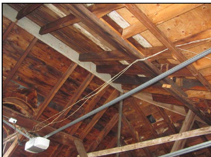
Photo No. 2: Garage roof rafters
