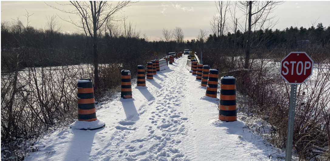
Figure 1: Additional stop signs and pylons installed at Elbow Creek Bridge
