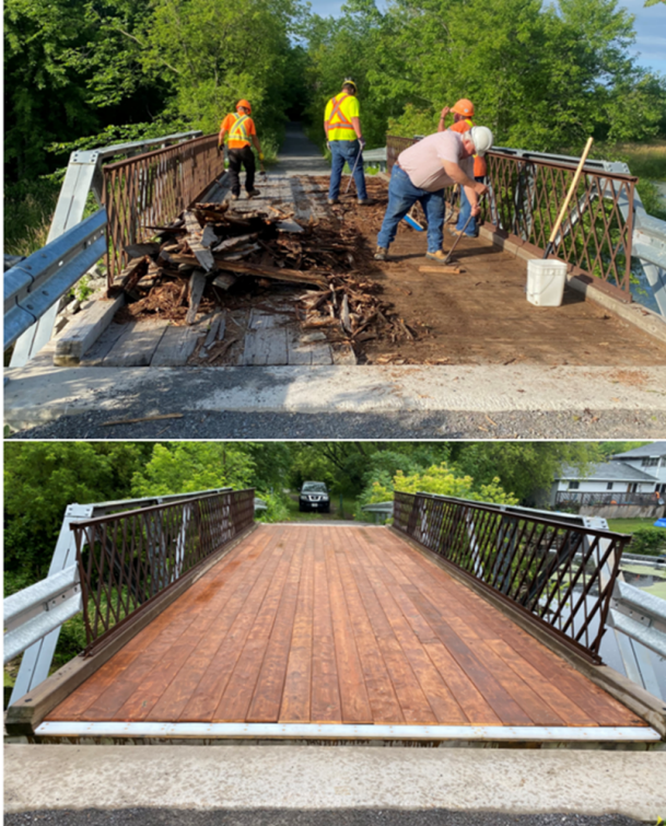
Figure 9 Hardwood Creek Bridge – before and after remediation
