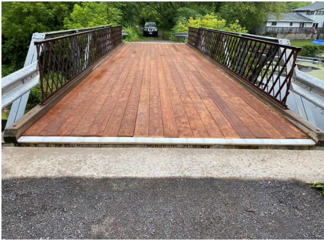
Figure 3 Hardwood Creek Bridge
