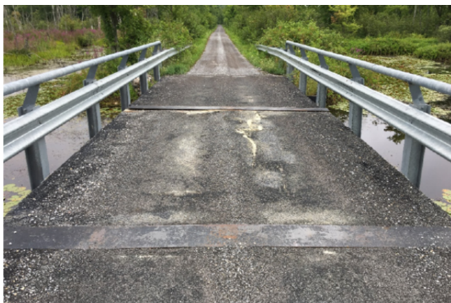
Figure 11 Elbow Creek Bridge
