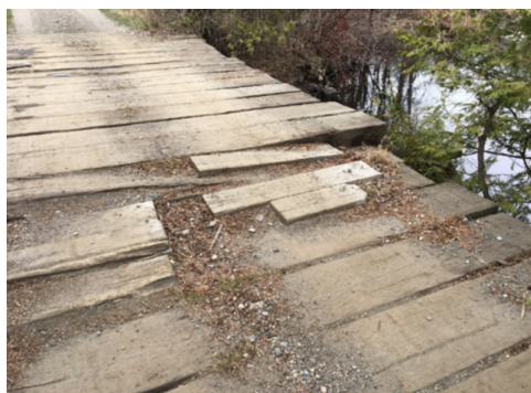
Figure 6 Bolton Creek 85-435 Mill Pond Bridge before remediation
