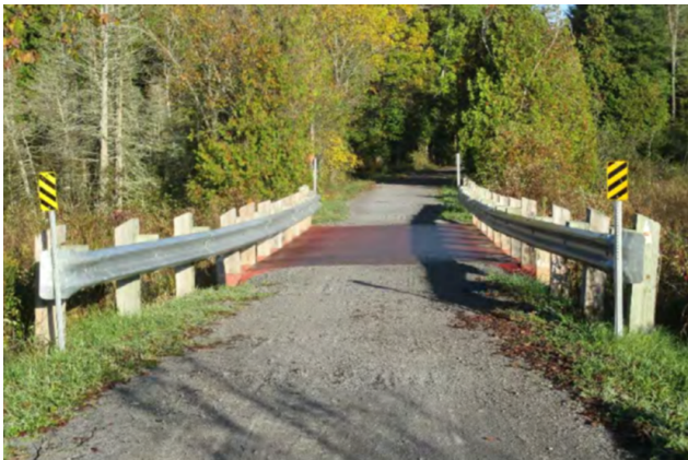
Figure 2 Millhaven Creek Bridge
