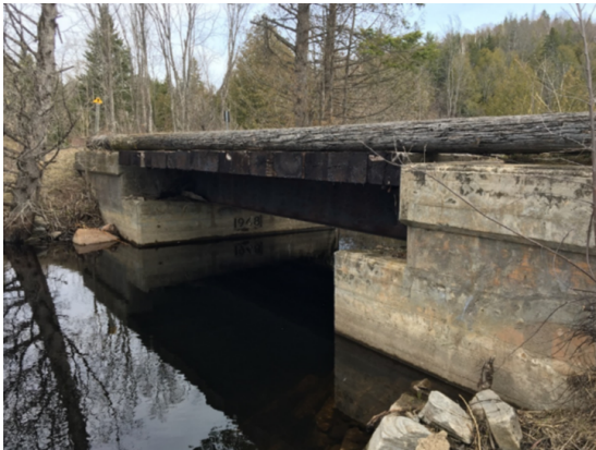
Figure 7 Bolton Creek Bridge North 86-015
