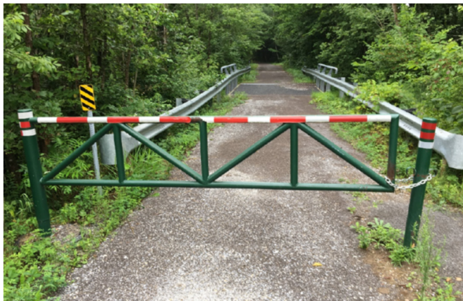
Figure 8 Fish Creek Bridge
