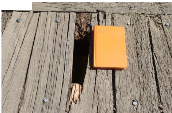
SW deck surface damage
