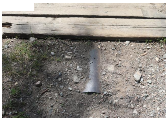
NW uncovered pipe girder
