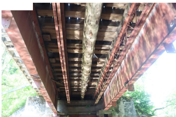
West wood spacer crushing
