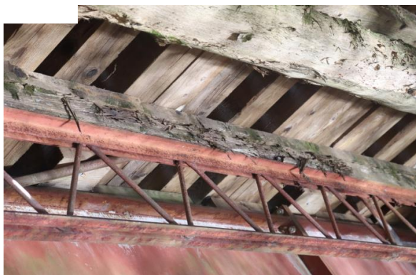
West wood spacer crushing
