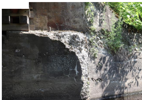
SE wing wall leaching & scaling
