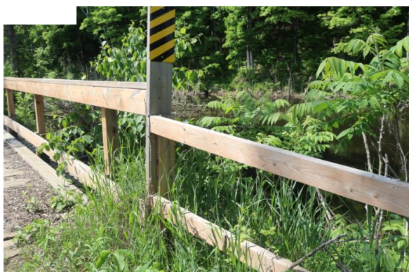
Approach rail - bridge rail connection
