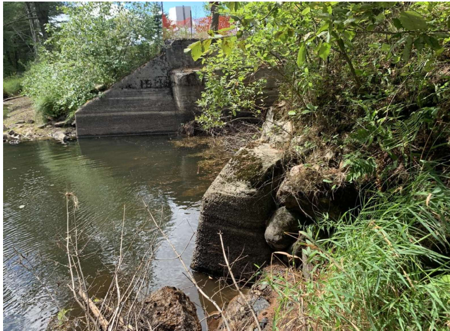
Figure 4 – Typical Wingwall with 1911 construction date (southeast shown)
