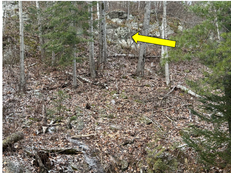
Photo 4 Existing Slope Face and Bedrock Cliff/Ledge Adjacent to Proposed Bunkhouse Location
