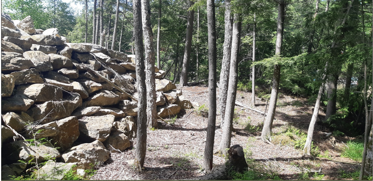
Figure 2: Photo showing the retaining wall on the subject property.
