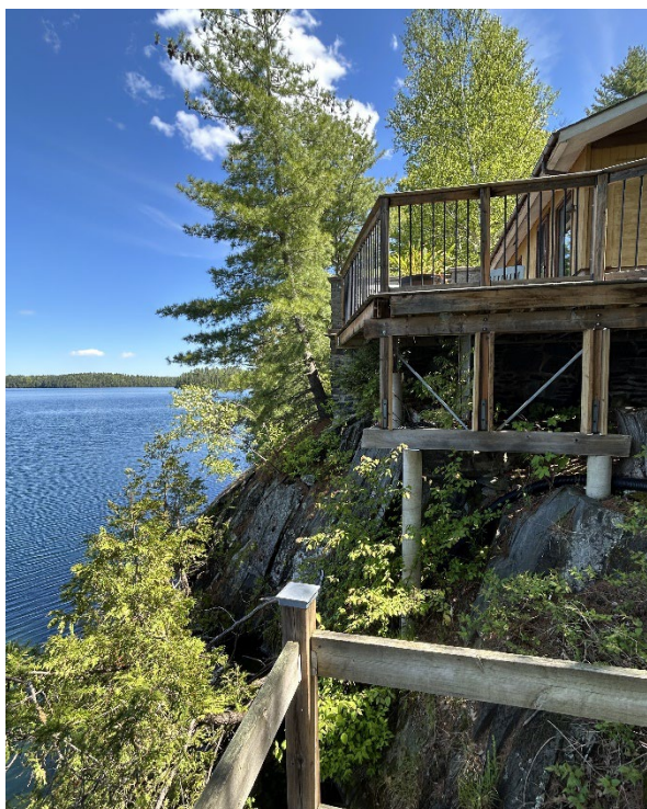
Photo 6 Slope Overview, West Side of Existing Dwelling, Facing East. May 2025.
