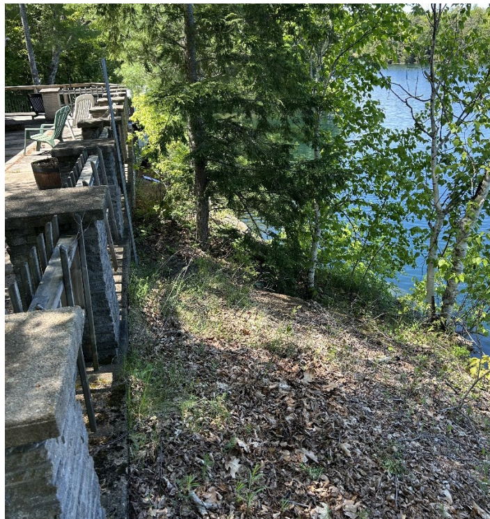
Photo 2 Slope Crest, North Side of Existing Dwelling, Facing West . May 2025.
