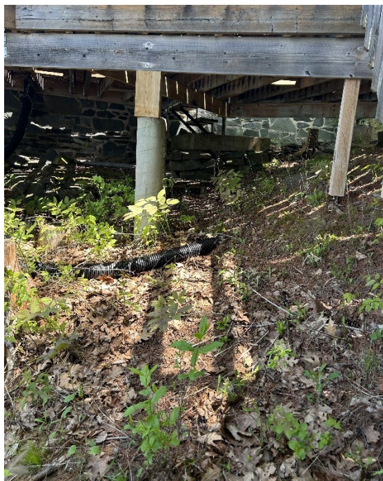
Photo 3 Slope Crest, West Side of Existing Dwelling, Facing East. May 2025.
