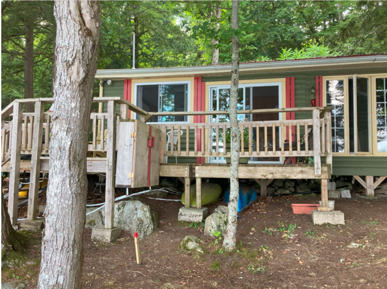
Figure 2: A focused picture of the where the proposed sunroom will be located in terms of the current deck layout.
