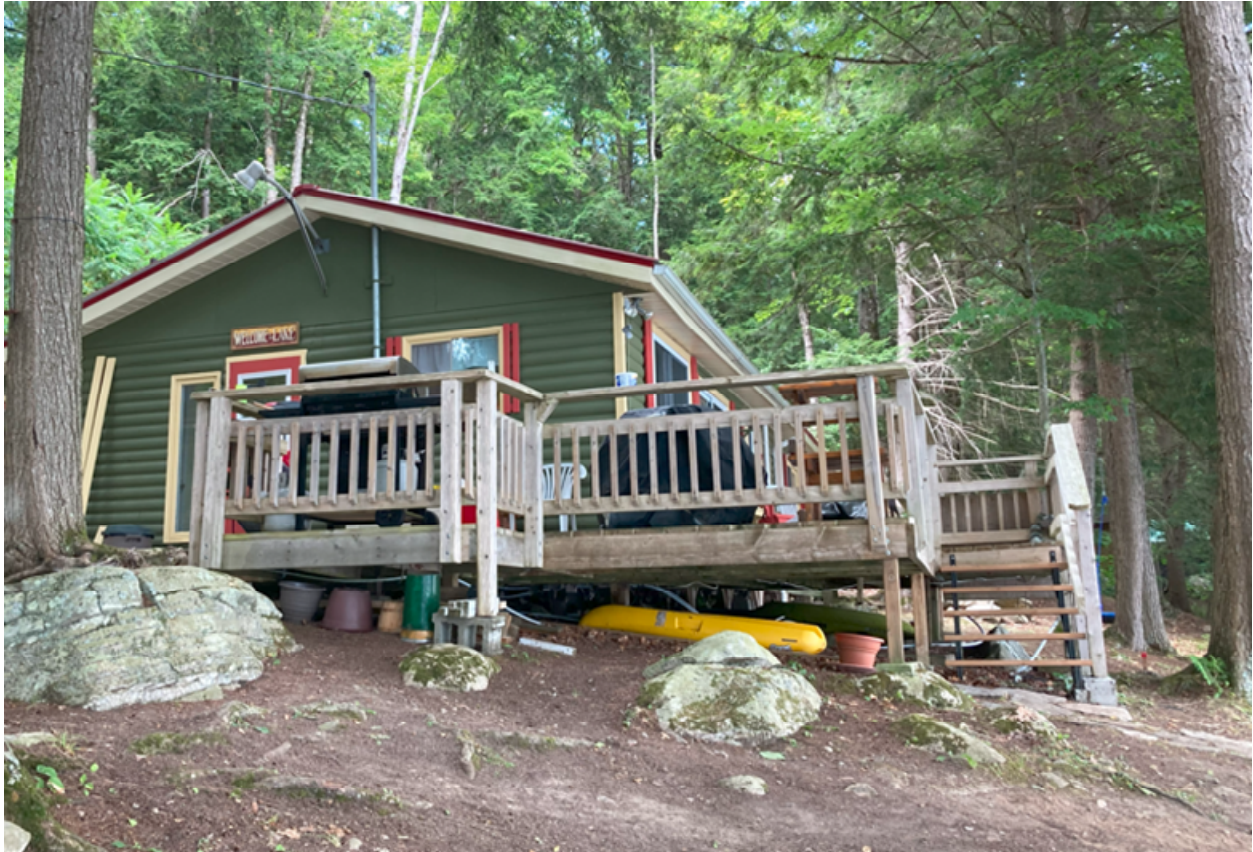
Figure 1: Picture of the current dwelling and deck from the west side.
