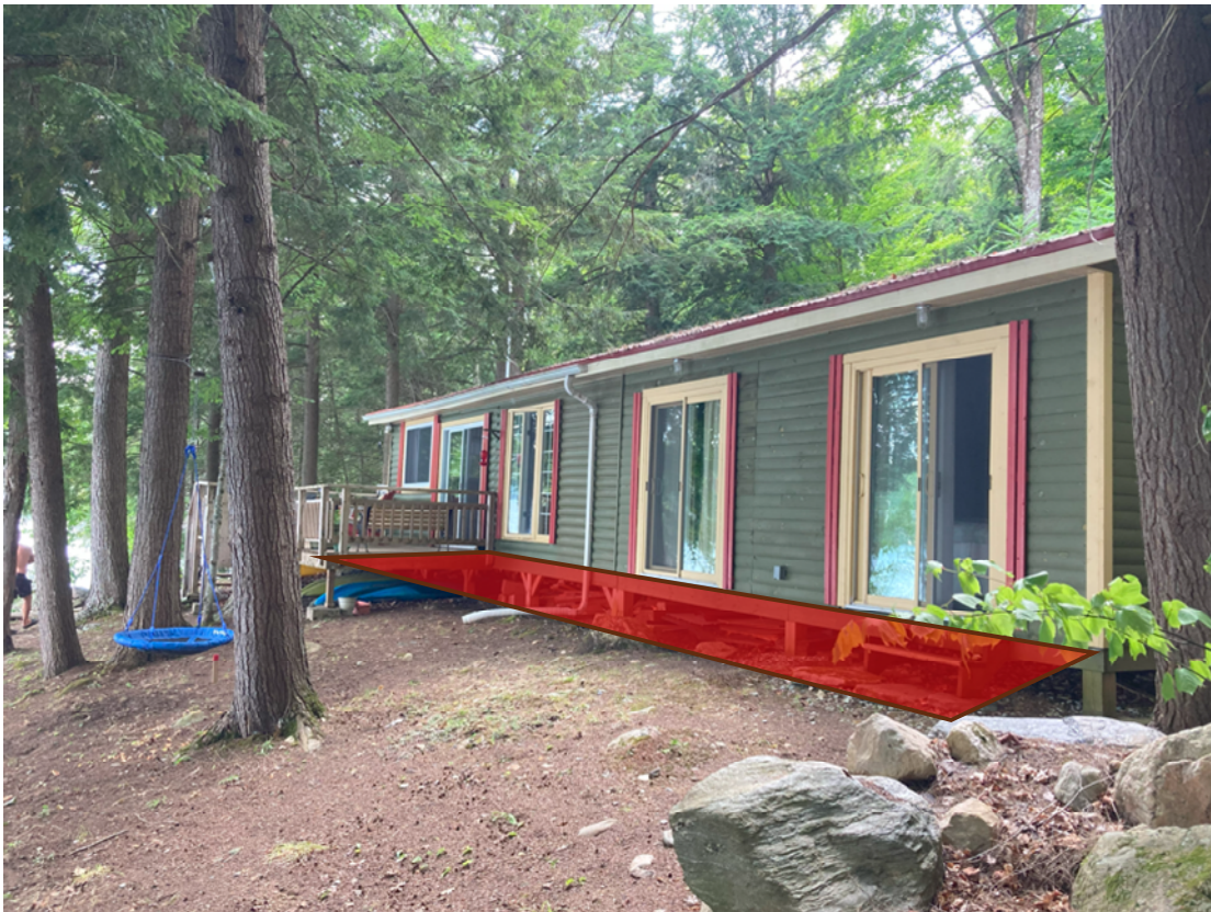
Figure 1. Image of the east side of the dwelling showing the location of the former deck in red.
