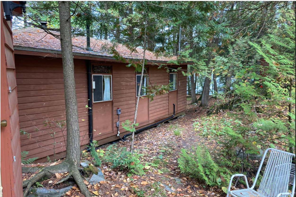
Figure 2. Area behind the existing dwelling proposed for addition
