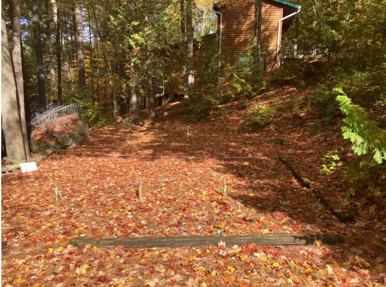
Figure 4. A closer shot of the flat area north of the dwelling. The stakes were placed by the applicant's septic installer prior to the submission of this application. It identifies the estimated locations of the distribution pipes.
