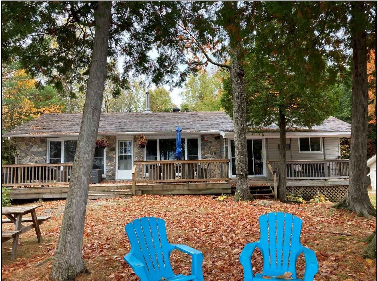
Figure 3: Image of the water side of the dwelling where the new screen porch will be located. The central section of railings is where the screen porch will be located.
