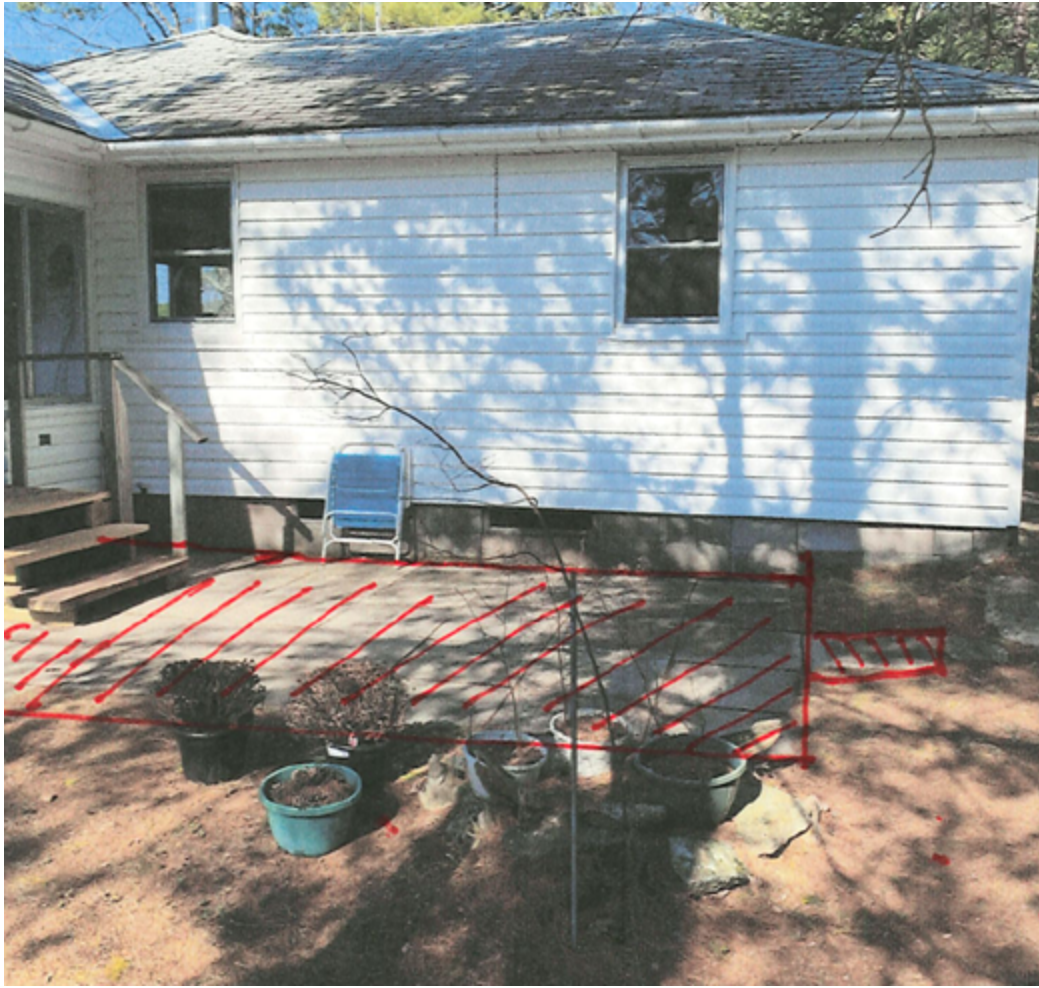
Figure 3. Image submitted with the application showing the state of the southwestern portion of the dwelling prior to construction.
