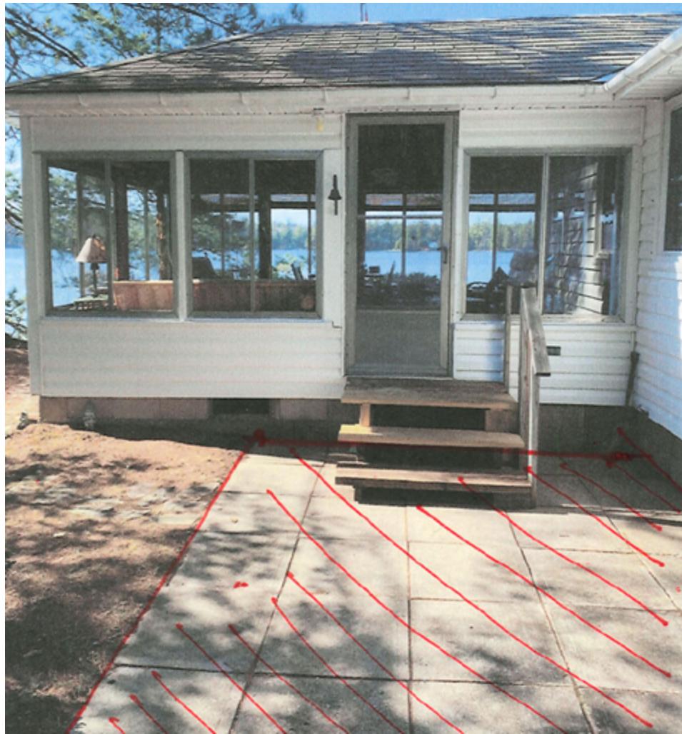
Figure 2. Image submitted with the application showing the state of the southwestern portion of the dwelling prior to construction.
