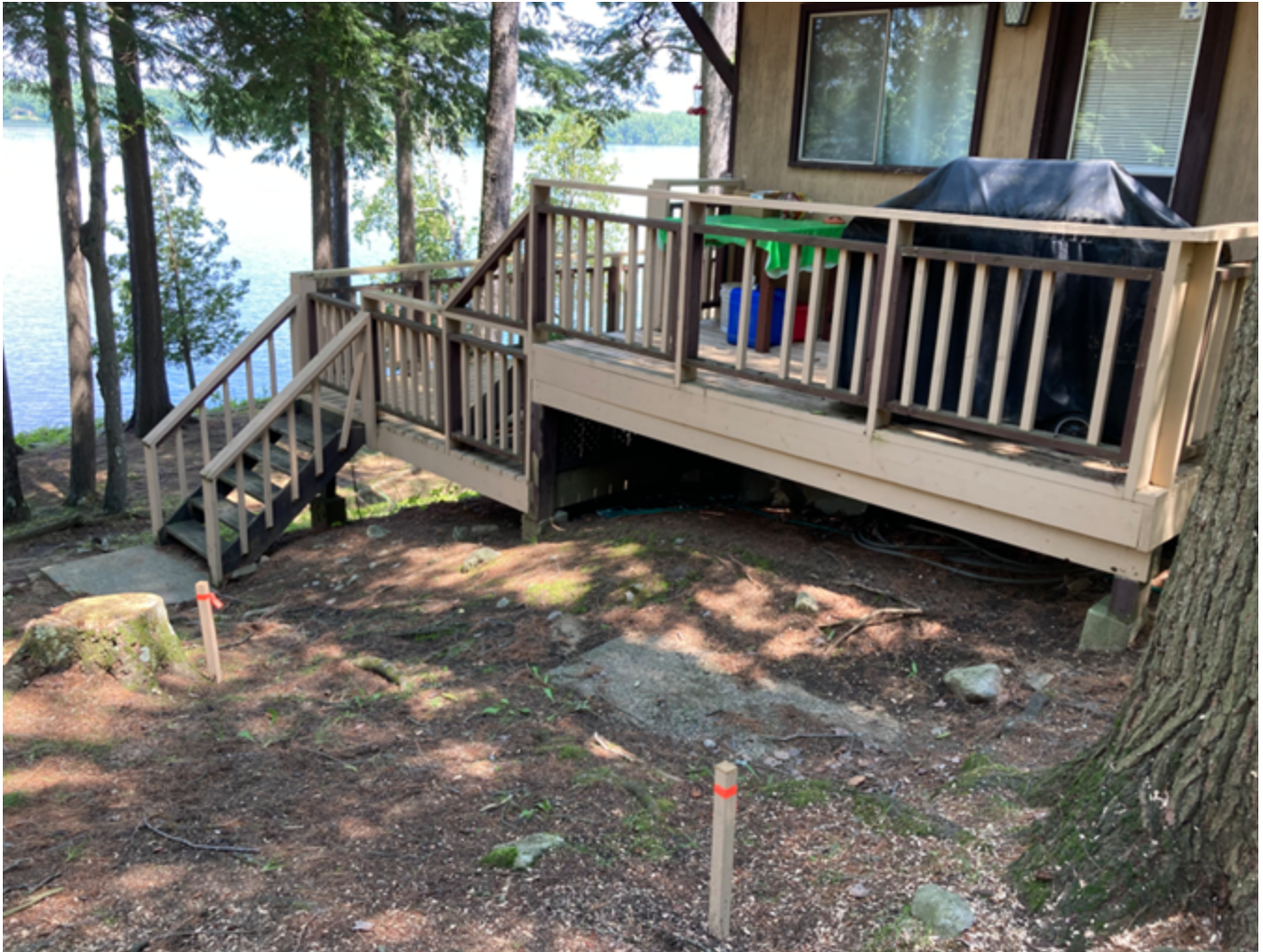
Figure 1. A photo of the proposed deck expansion area. The stakes show the extend of the deck expansion.
