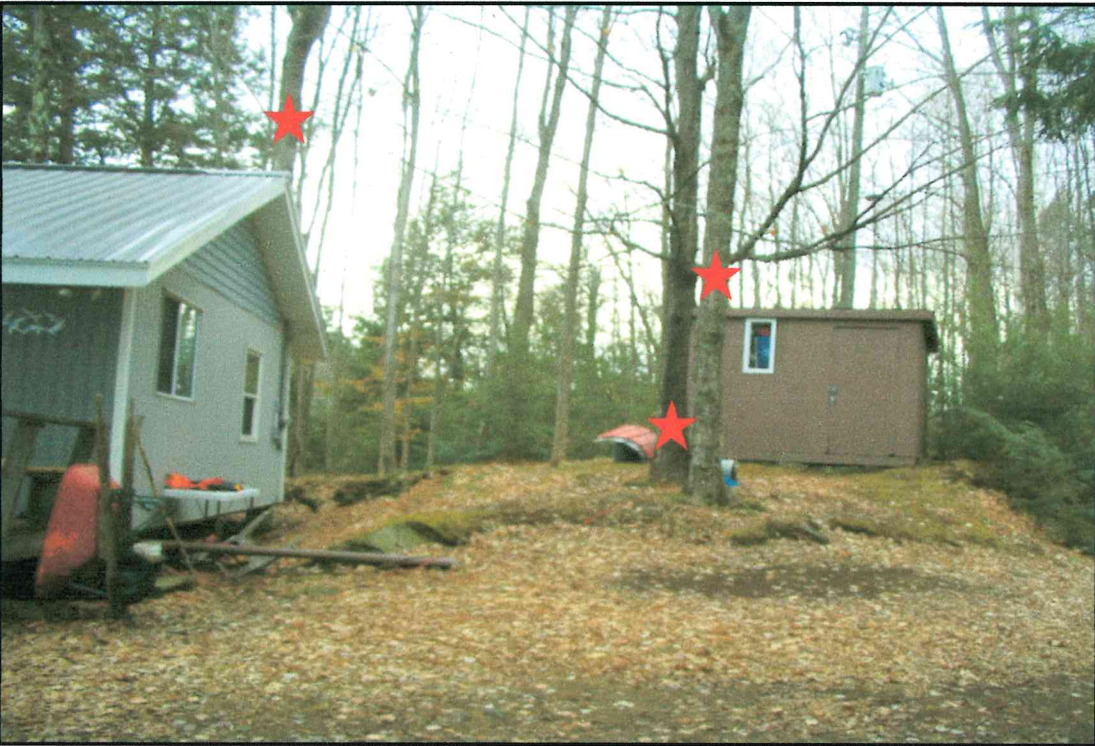
Photograph 2 – View of North end of Cottage where addition is proposed – Shows Natural Grade and trees to be removed
