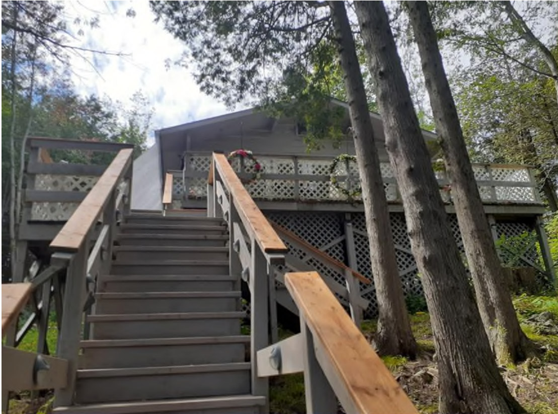
View from bottom of deck
