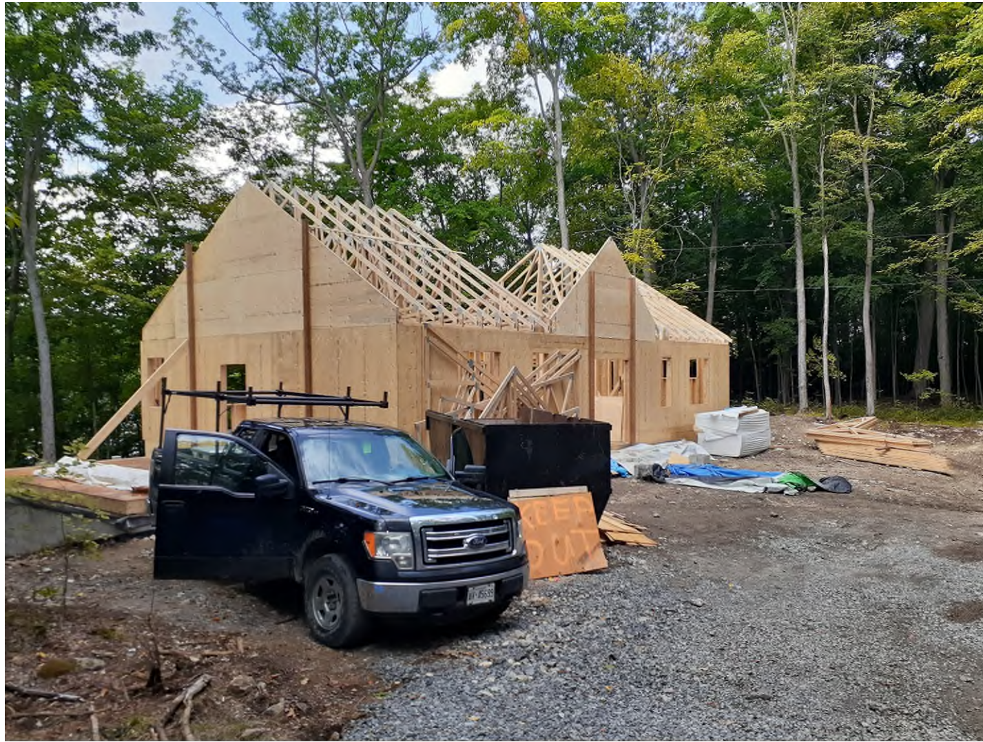
Seasonal dwelling under construction
