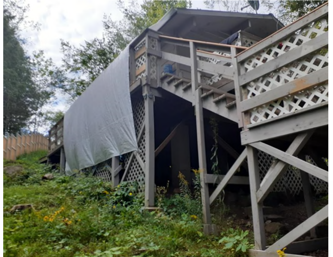
View of the cement blocks under house
