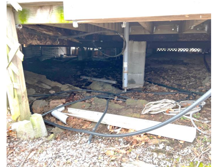
Photo 3 Pier foundations of existing residence placed directly on bedrock.
