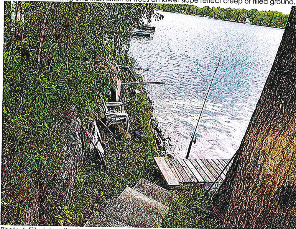
Photo 4 Filled shoreline beyond outcropping bedrock. It is understood the cottage dates from the 1950s.
