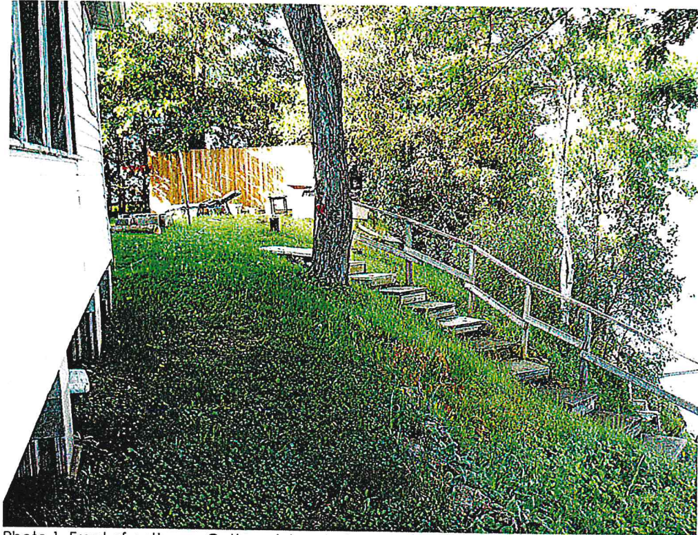
Photo 1 Front of cottage. Cottage is located on a terrace defined by shallow marble bedrock.
