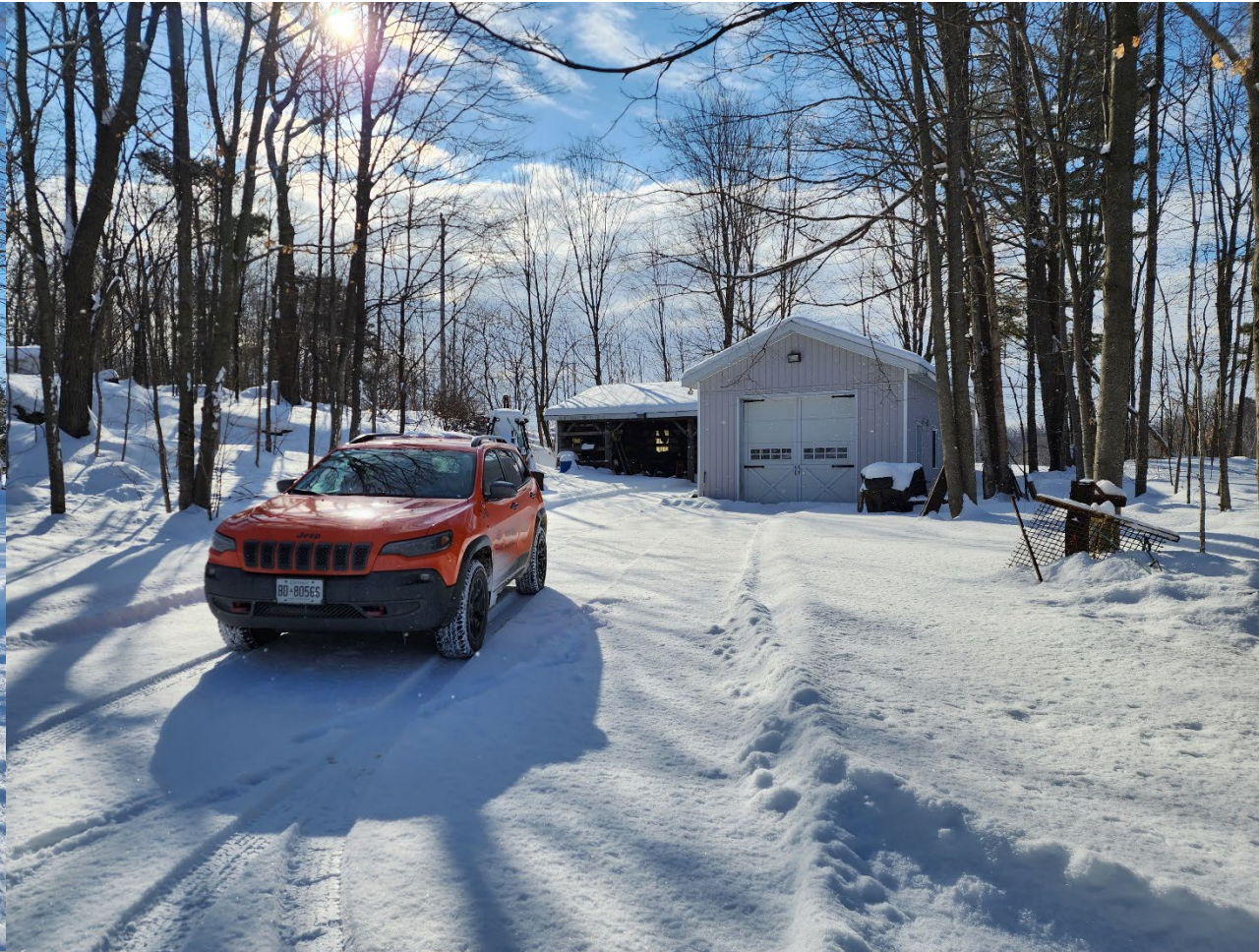
Subject Property – Existing detached garage
