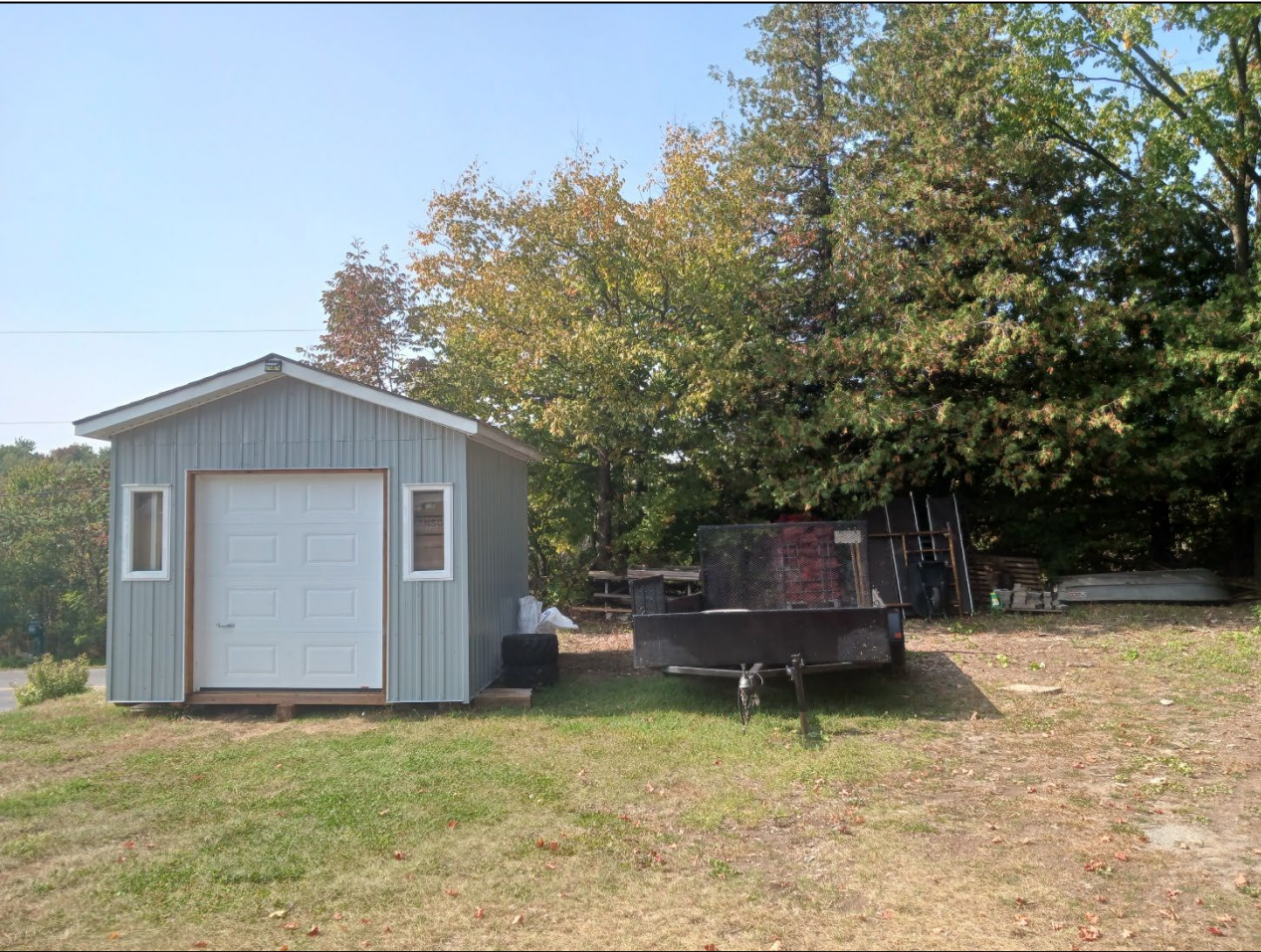
Location of existing & proposed structures (Facing east towards Holleford Road)
