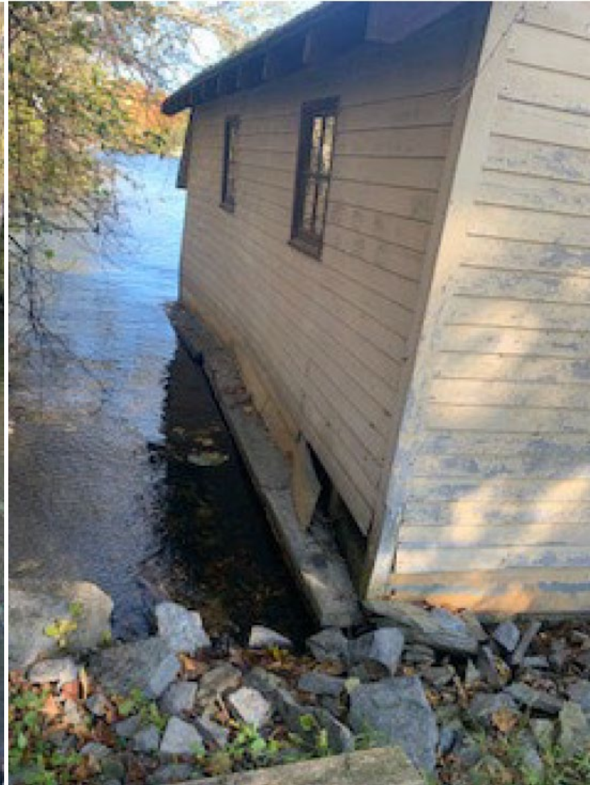
Along west side
