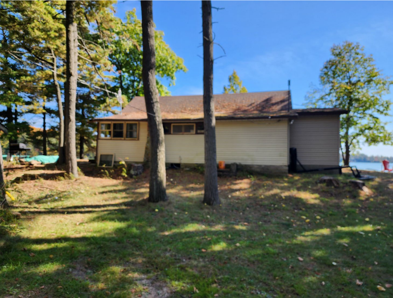
North side of dwelling
