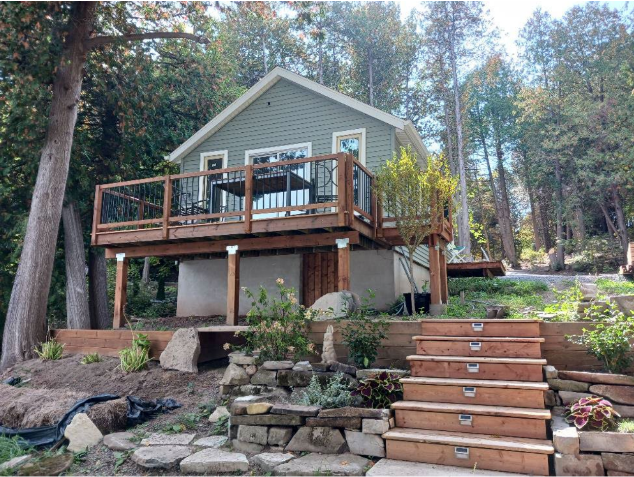
Existing seasonal dwelling (front view)
