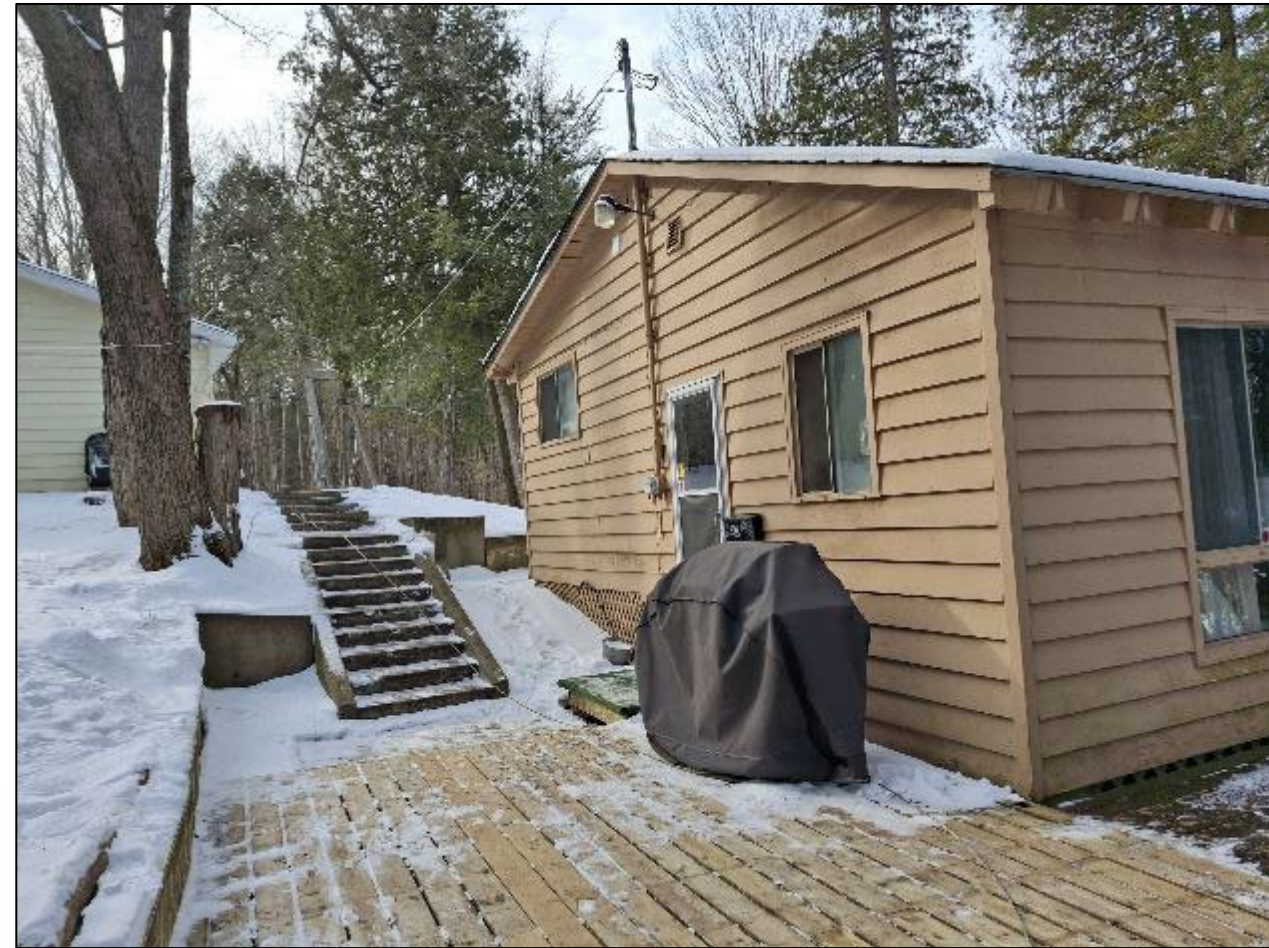
Existing Dwelling (Side View)
