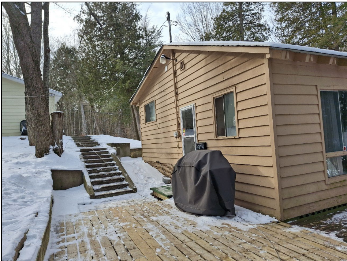
Photo 4 – Existing side deck (location of proposed screened porch addition)
