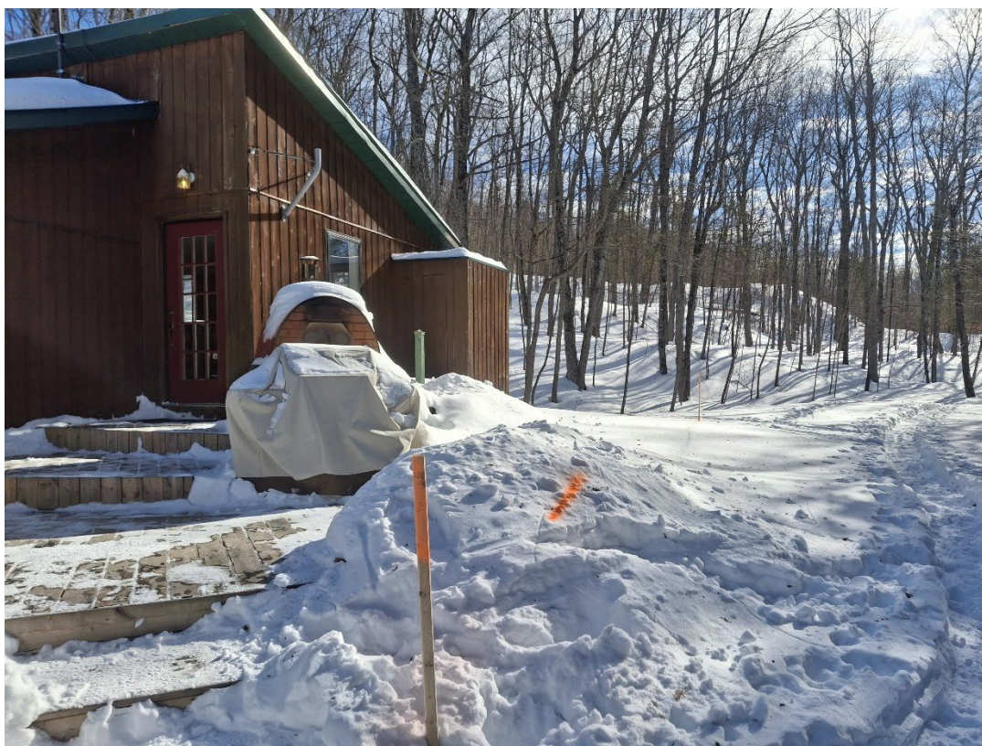
Photo 4 – West side (location of proposed screened-in porch)
