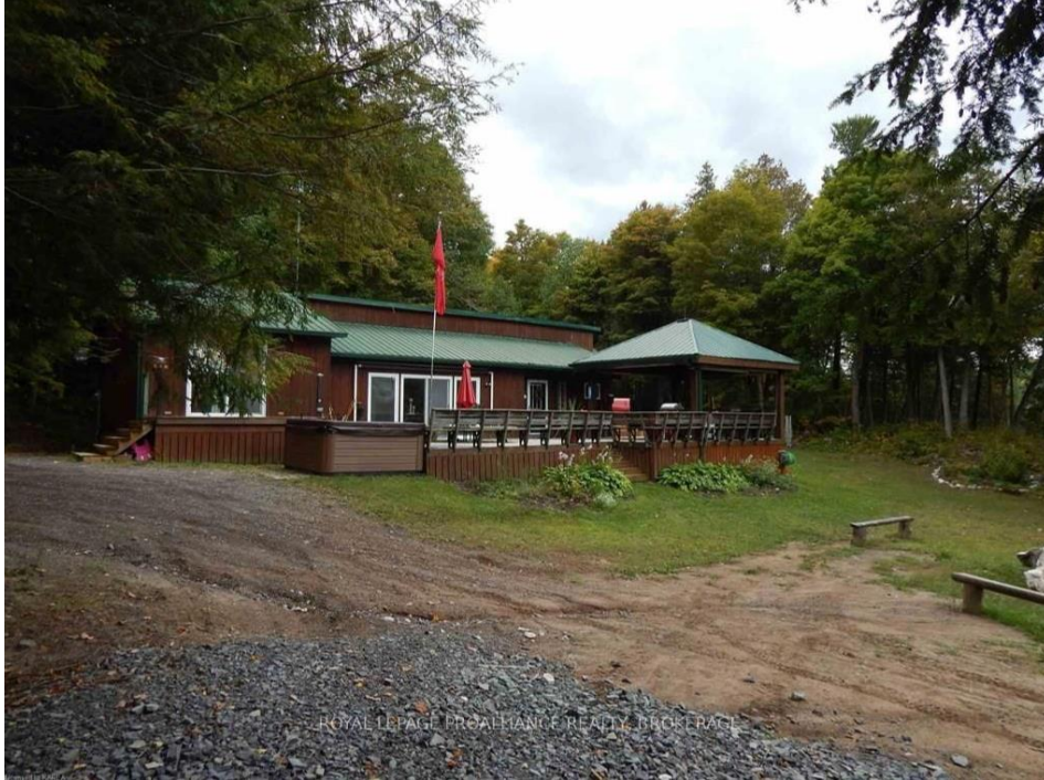
Image 1: Photo taken from waterfront side of property to show elevation of house. The large granite ridge can be seen on the right side of the image running along the side of the property
