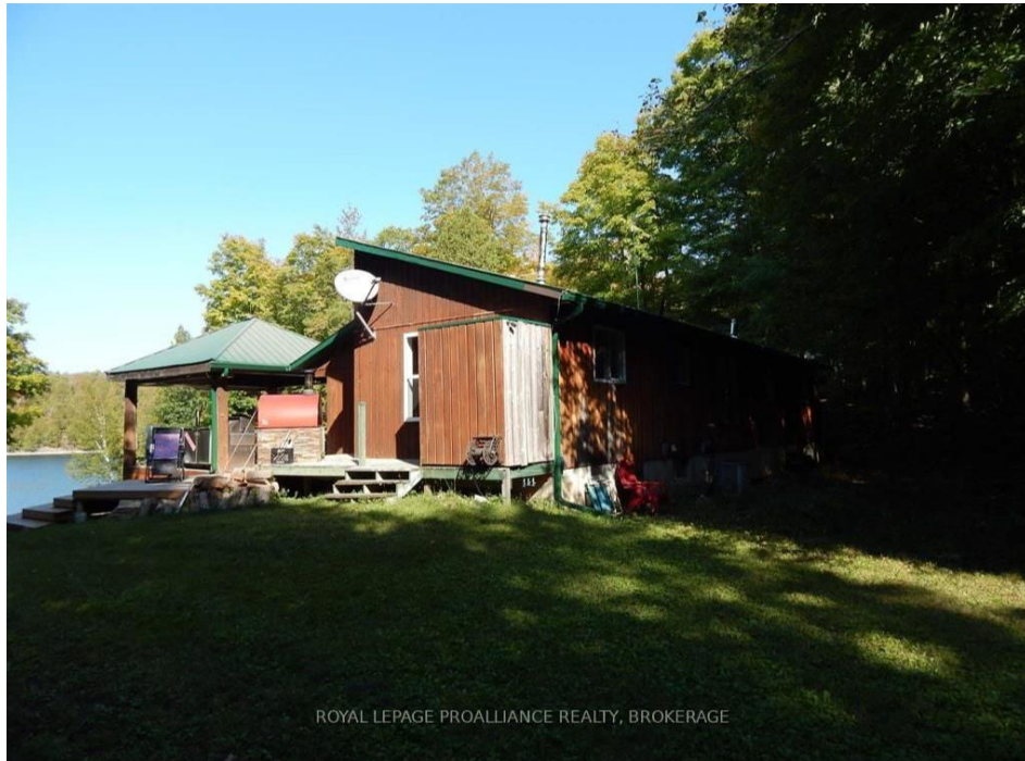
Image 3: View of existing west end of the house with current decks
