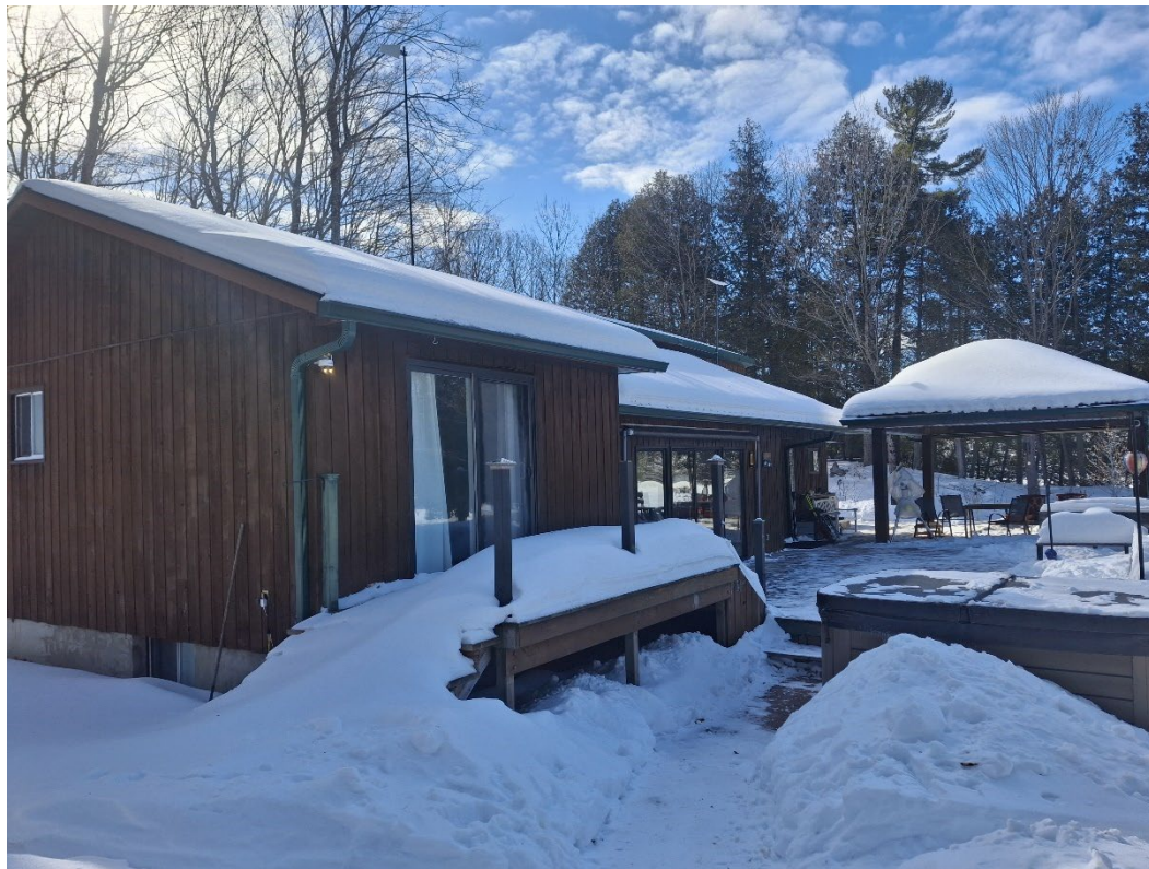
Photo 3 – Front view showing existing attached deck
