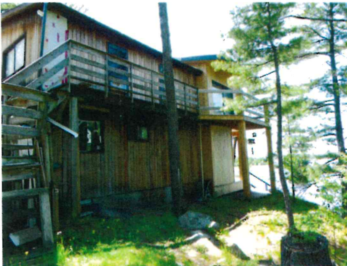
Photo 1. View to the west (Dog Lake in the distance). The lighter wood of the rebuild/addition can be seen to be sitting on bare rock. Note the sparse ground vegetation. 2016.05.23.
