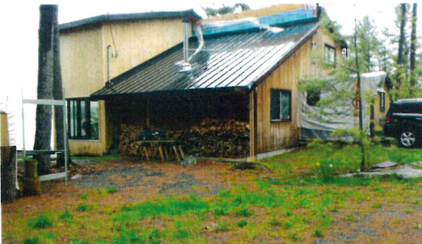
Photo 7. View to the NNW at the end of the cottage where the proposed addition will go, encompassing the tarp-wrapped Frame Deck, and continuing in line with the existing structure, and including a carport over the gravel drive. Note the sparse lawn and gravel-treated substrate, and the young White Pine that will be removed or relocated. 2016.05.13.
