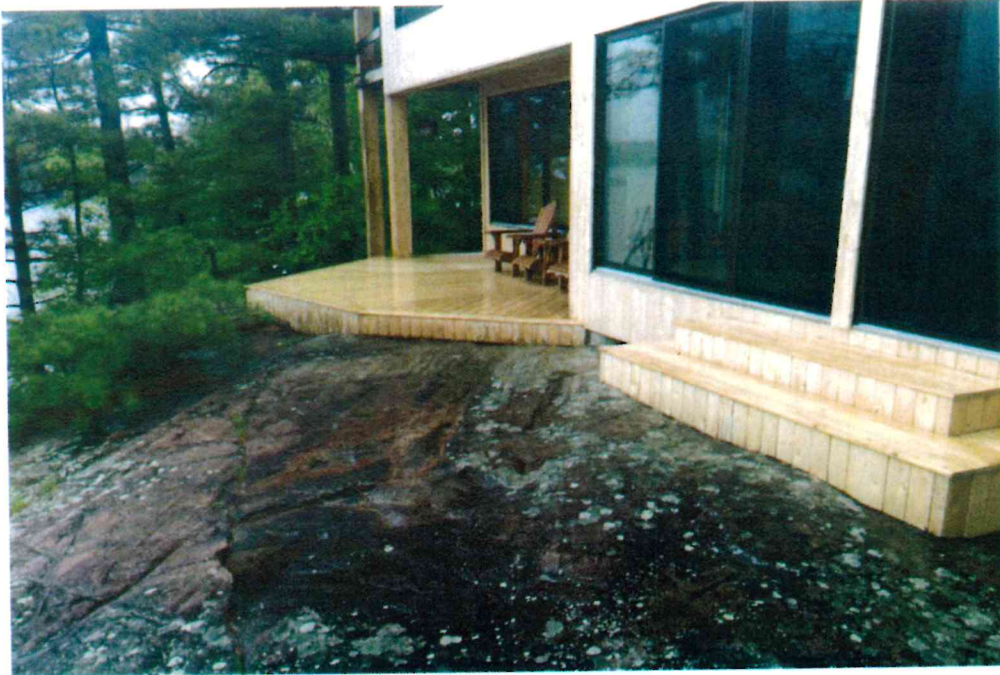
New Addition – looking north
