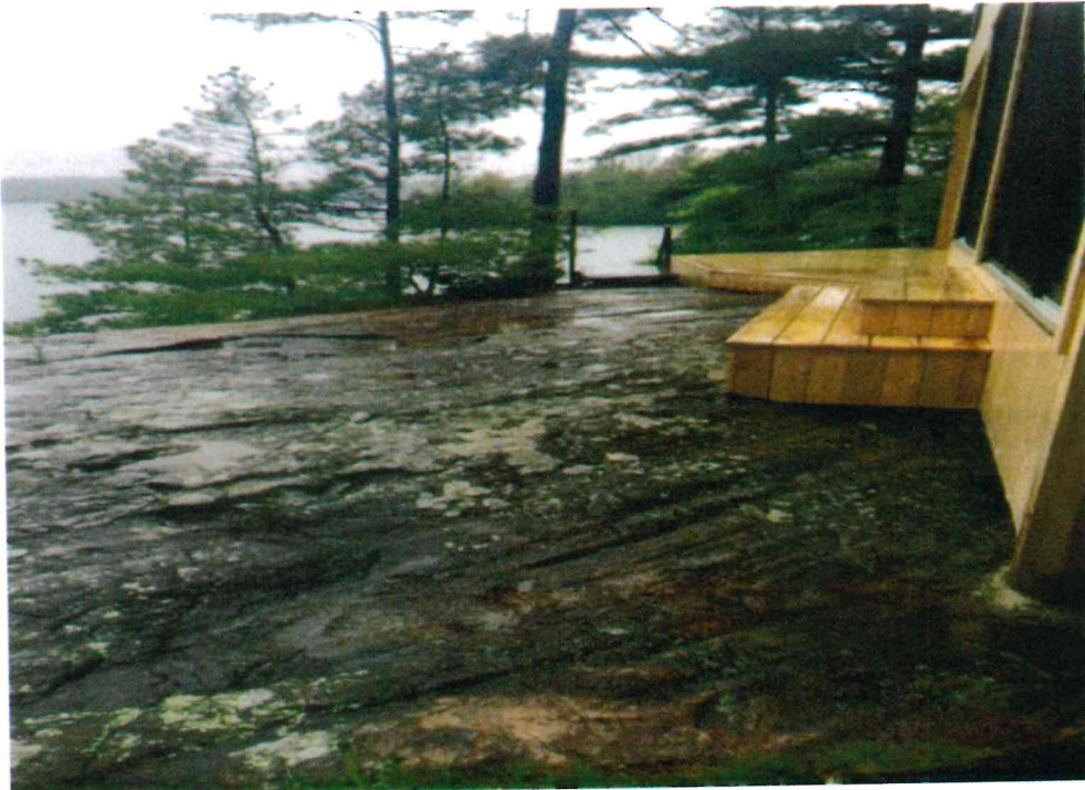
New Addition – looking north
