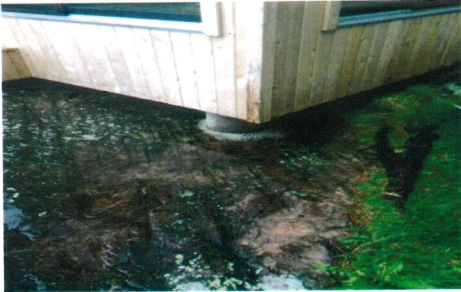
Typical footing – new addition
