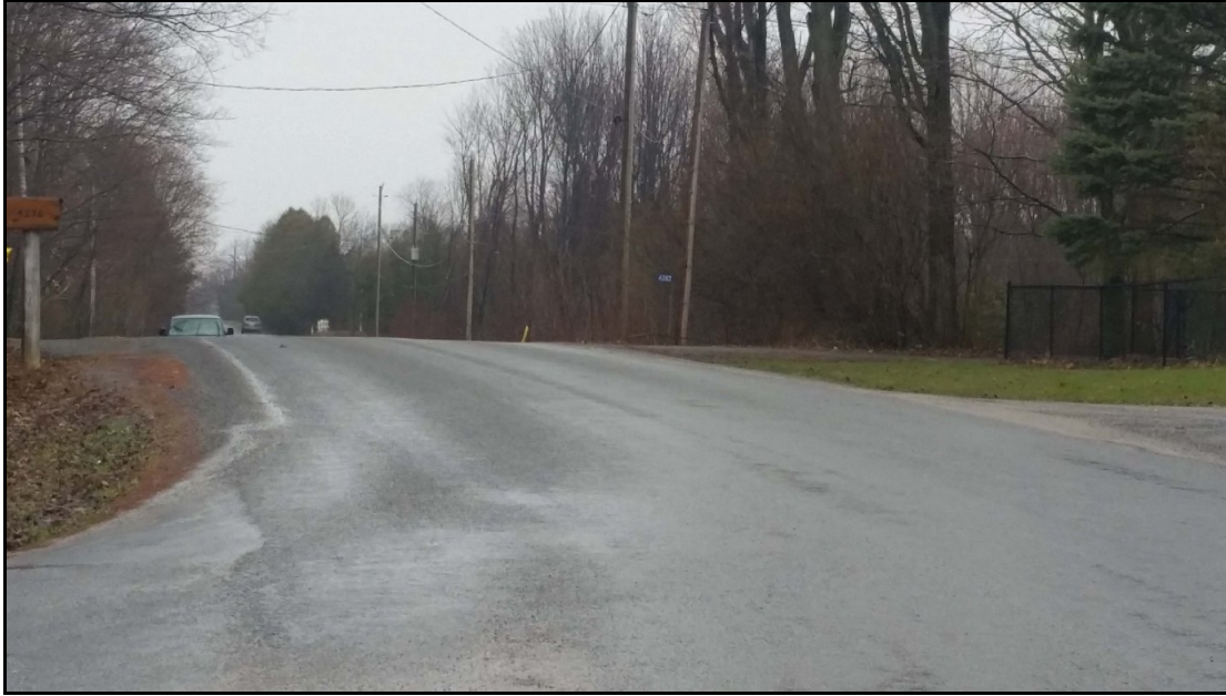
Plate 3: Looking west on Holmes Road from the intersection with Lakefield Drive. The full-sized van is almost complete obscured by the hill, yet is approximately 50 metres from the intersection. Any accident in this area will completely cut off residents within Lyon's Landing - a problem that will be exacerbated by any additional development.
