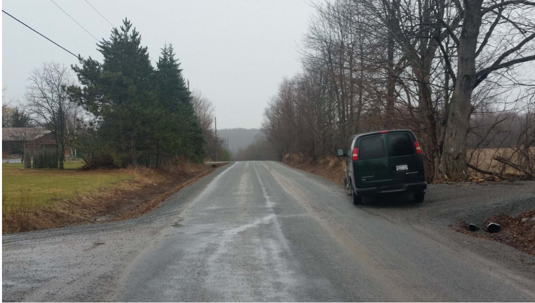
Plate 5: View from the intersection of Maple Crest Court and Lakefield Drive looking south. Traffic proceeding north up the steep hill towards Maple Crest is invisible until they breast the rise. The addition of another road and additional traffic at this location will add to an already dangerous intersection.
