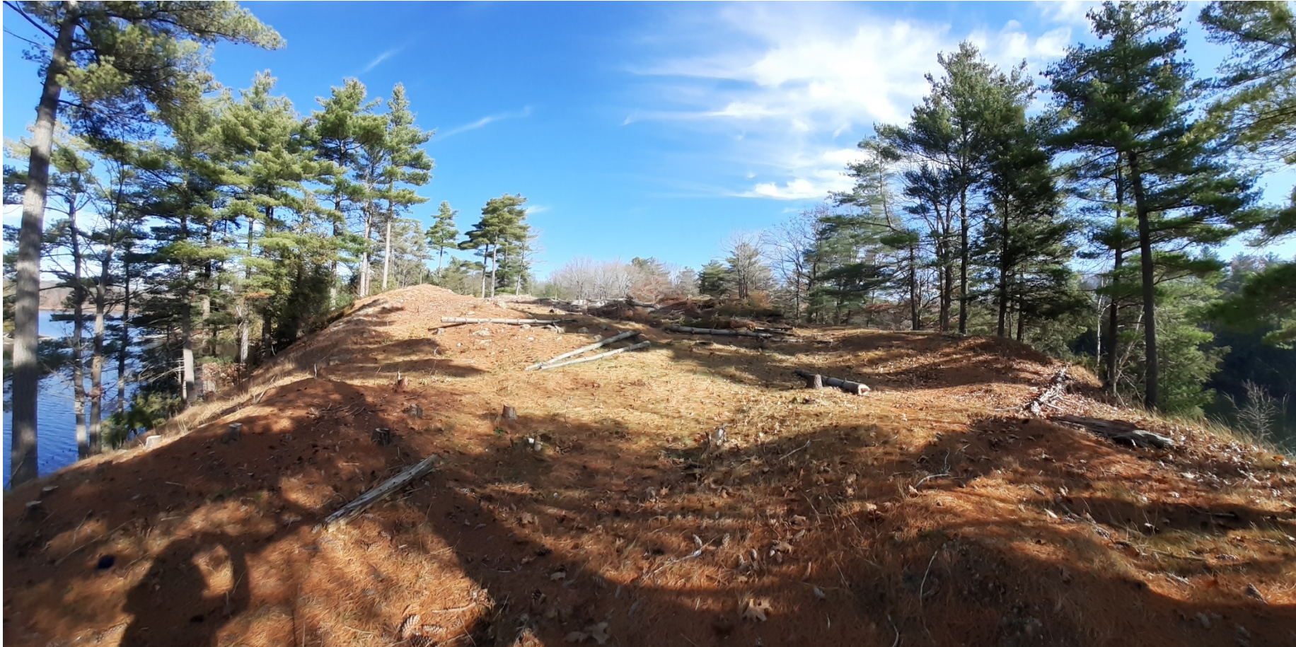
Looking north – sewage system in foreground, house in background
