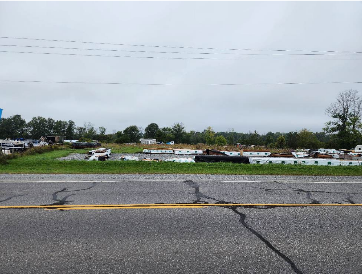
Towards area of new building supply outlet and new entrance
