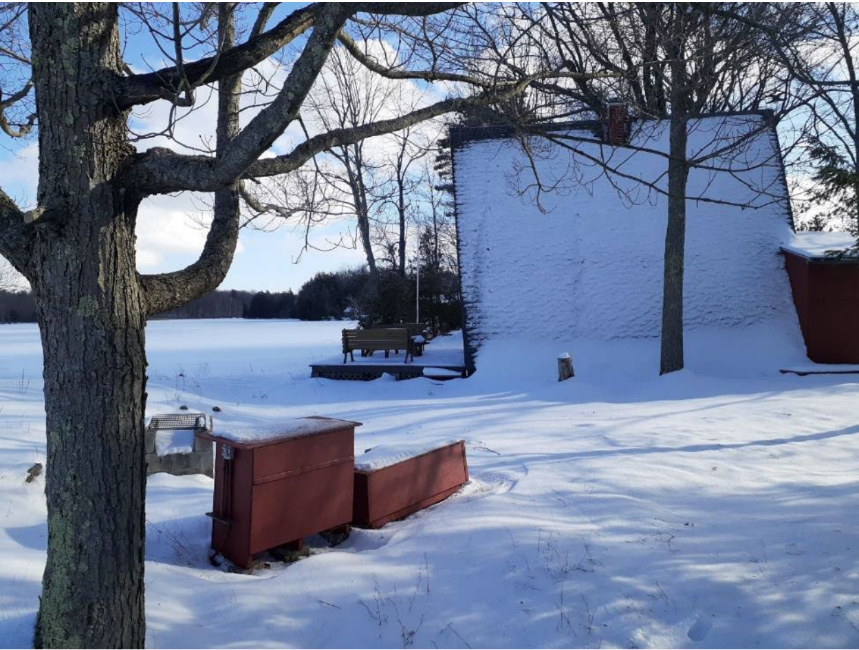
Existing cottage relative to shoreline
